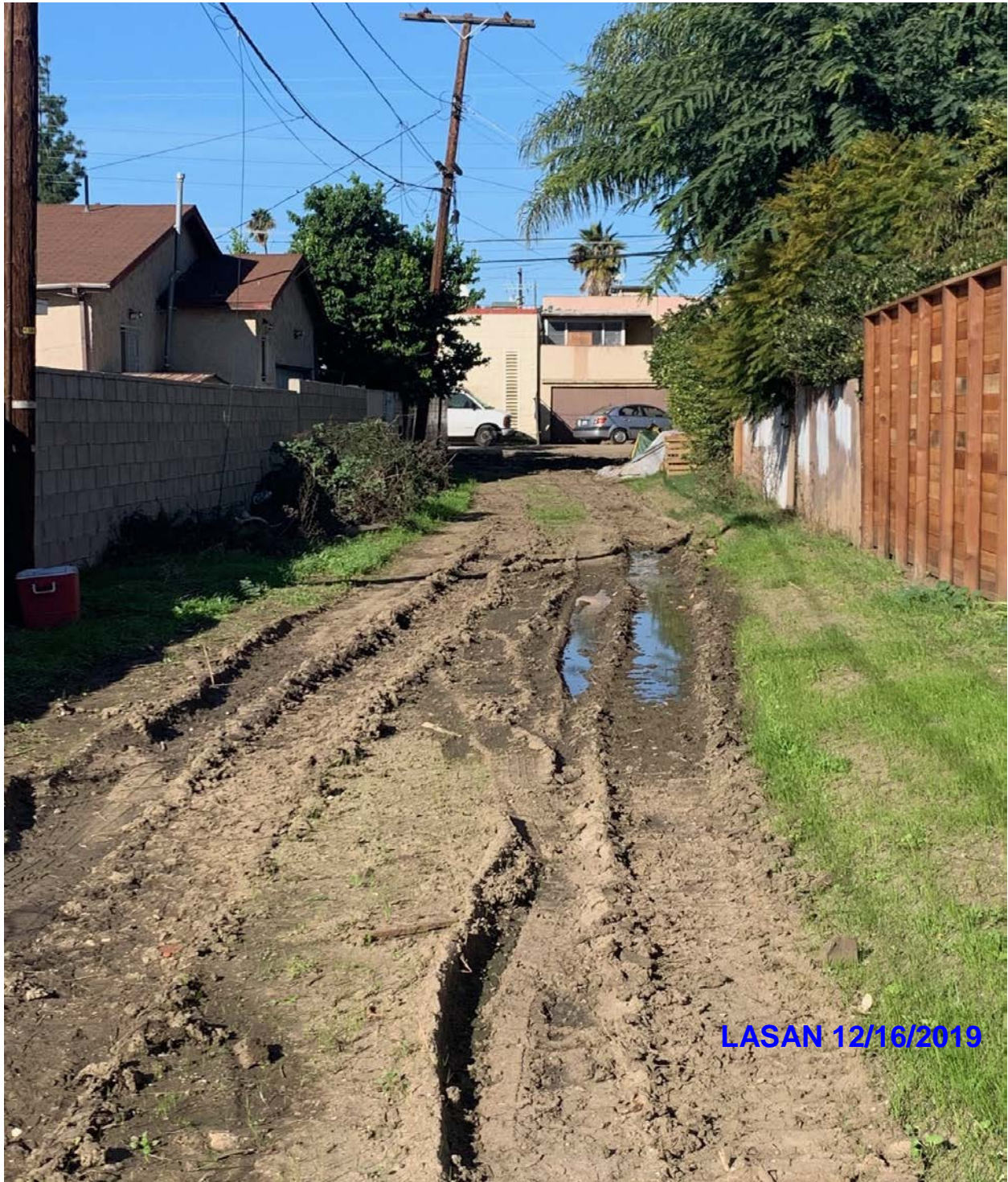
Figure 2. Condition of unimproved alley after storm: tread marks, mud and ponding
