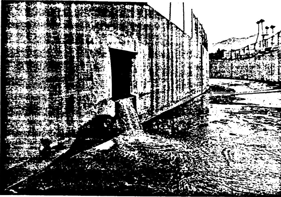
Picture 2. Discharge at North Stable Outfall: showing small debris and accumulated sediment
