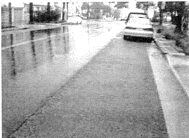
Figure 4: Permeable pavement during a storm event ( Model for Living Streets Design Manual, 2011 ).
