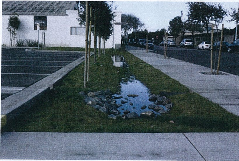
Figure 8: Vegetated swale (Signal Hill, CA).
