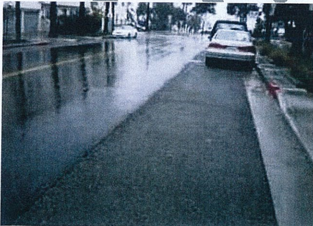
Figure 4: Permeable pavement during a storm event ( Model for Living Streets Design Manual, 2011 ).
