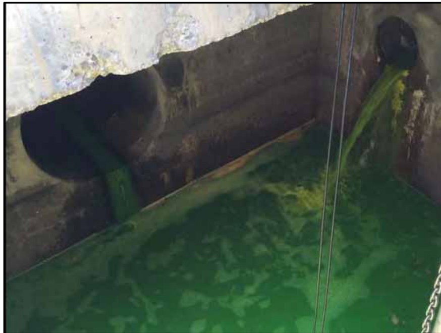
36" and 18" RCPs discharging to Pump Station Containment Vault (Provided by the County)
