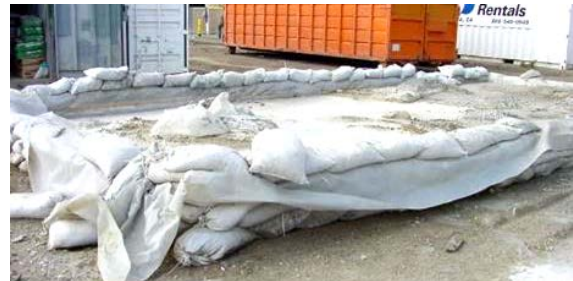
Concrete washout at construction site
