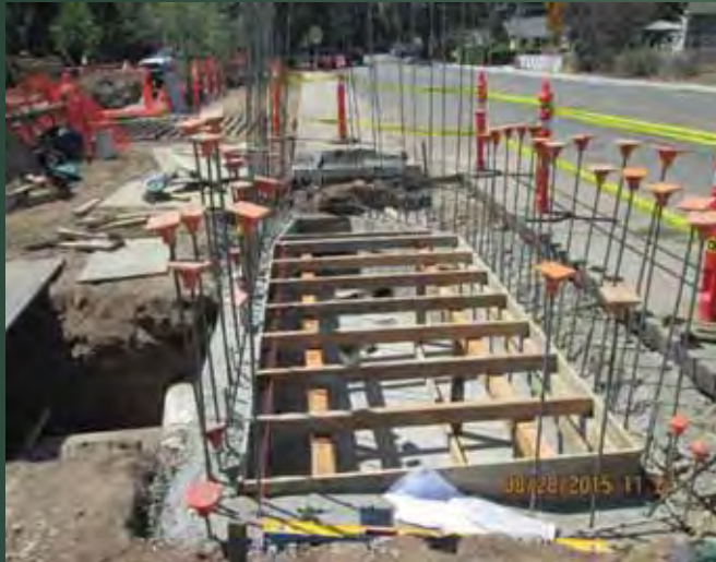
Concrete and forms for diversion catch basin and transition structure
