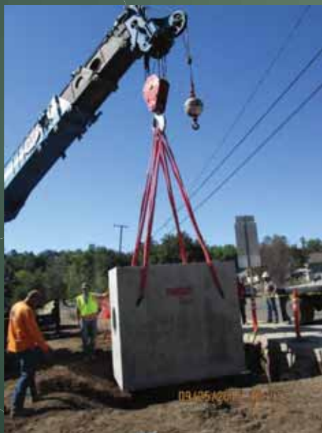
Baffle box vault placement
