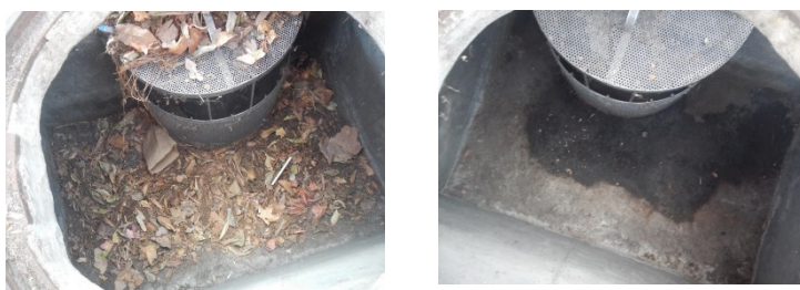
Full Capture Device Cleanout in October 2016.
