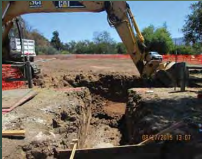
Excavation for treatment vault
