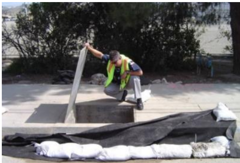
Inspection of catch basin BMPs
