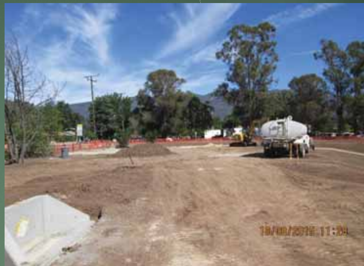
Concrete headwall for swale discharge piping
