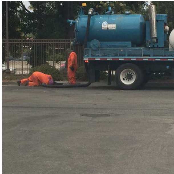
Catch Basin Cleaning Using a Vacuum Truck
