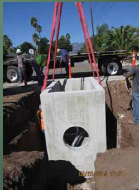
Baffle box vault placement
