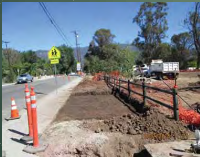
Excavated area for maintenance vehicle parking (out of traffic)
