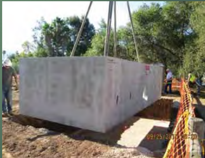
Treatment vault placement
