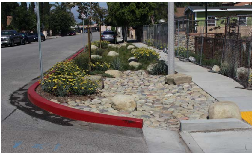
Low Impact Development infiltration BMP
