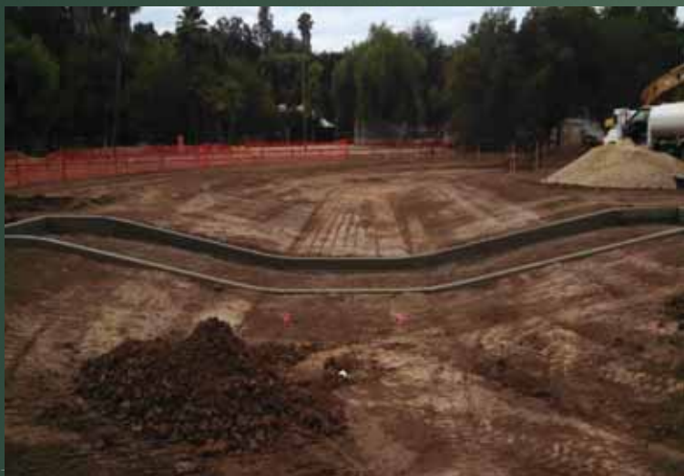
Graded swale and OVLC maintenance crossing
