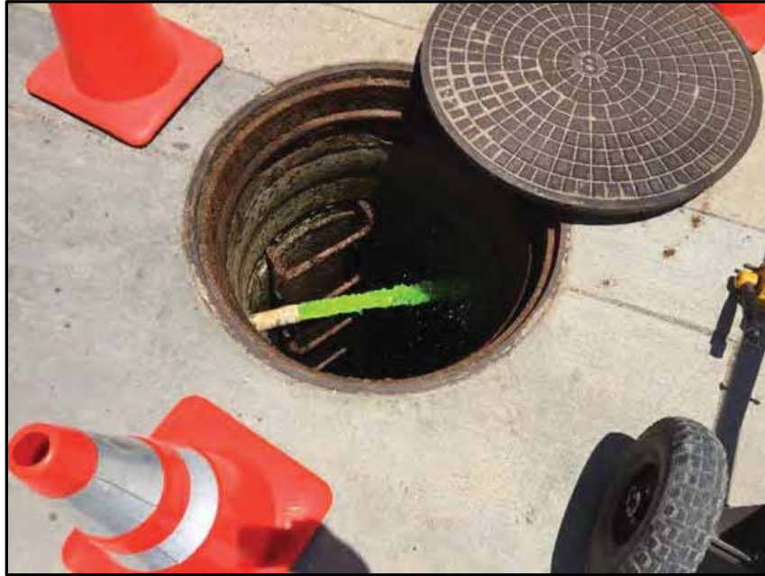
Sewer diversion pump discharging to sanitary sewer system (Provided by the County)
