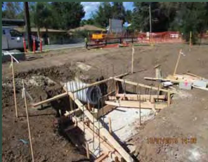
Constructing concrete headwall for swale discharge piping
