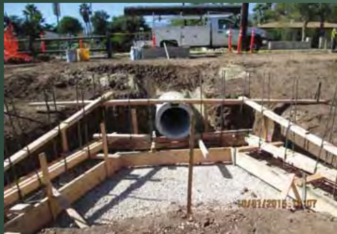
Constructing concrete headwall for swale inlet piping from baffle box
