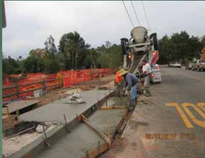
Diversion catch basin and inlet local depression concrete work
