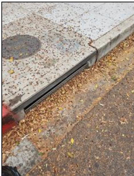
Figure 13. Catch basins along the study routes had curb screens that prevented trash from being swept into them.
