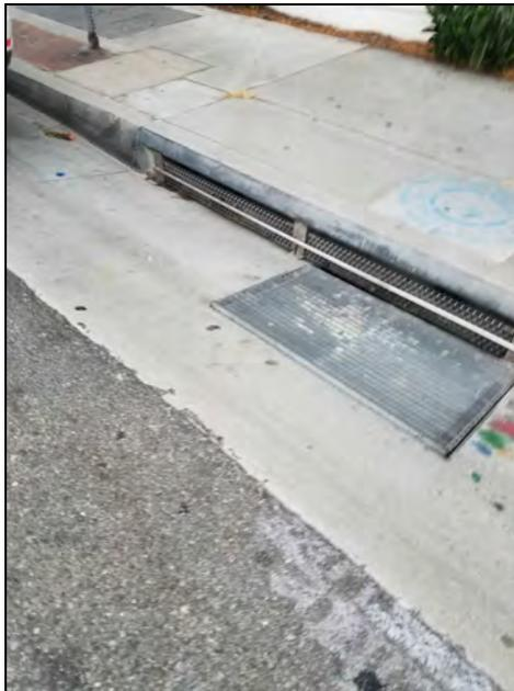
Figure 9. Catch basins along the study routes have curb screens to prevent trash from being swept into them.
