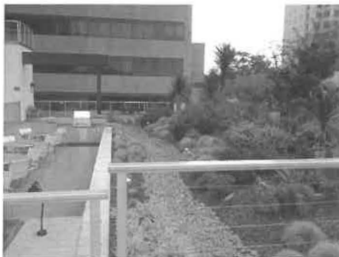
Bioretention system (Planter Boxes, City of Los Angeles)
