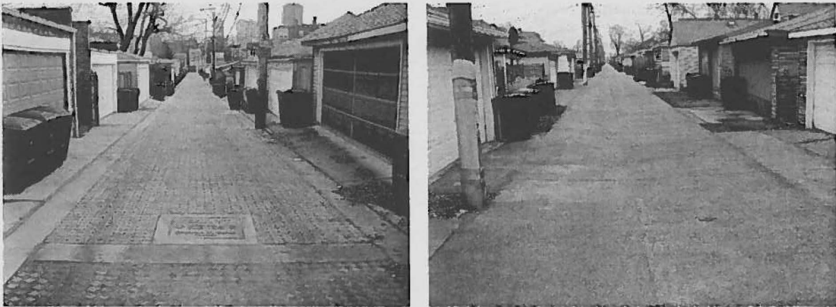
Figure 10: Permeable Pavers and Permeable Concrete Chicago Alleys (Source: Abby Hall, US EPA)
