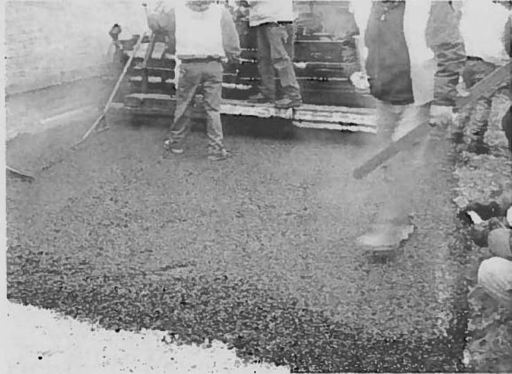
Figure 9: Permeable Asphalt Installation Using Ground Tire Rubber.
