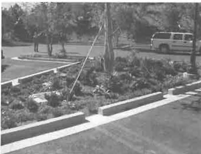
Bioretention in a parking lot (GeoSyntec)
