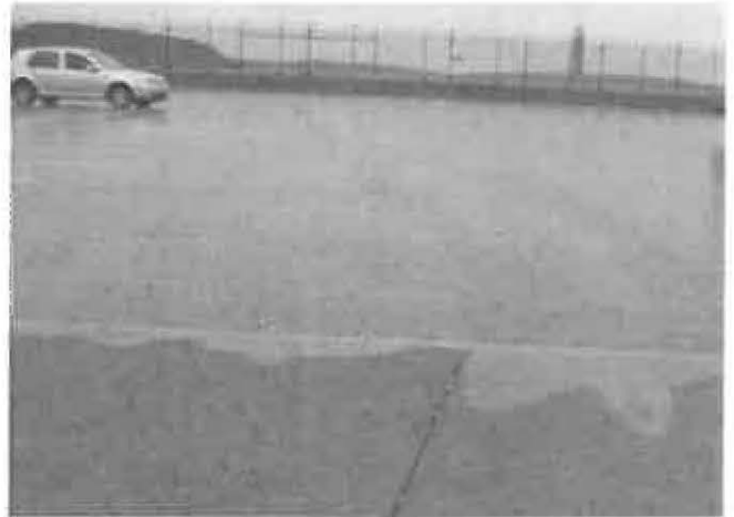
Permeable pavement, City of Los Angeles Airport parking lot
