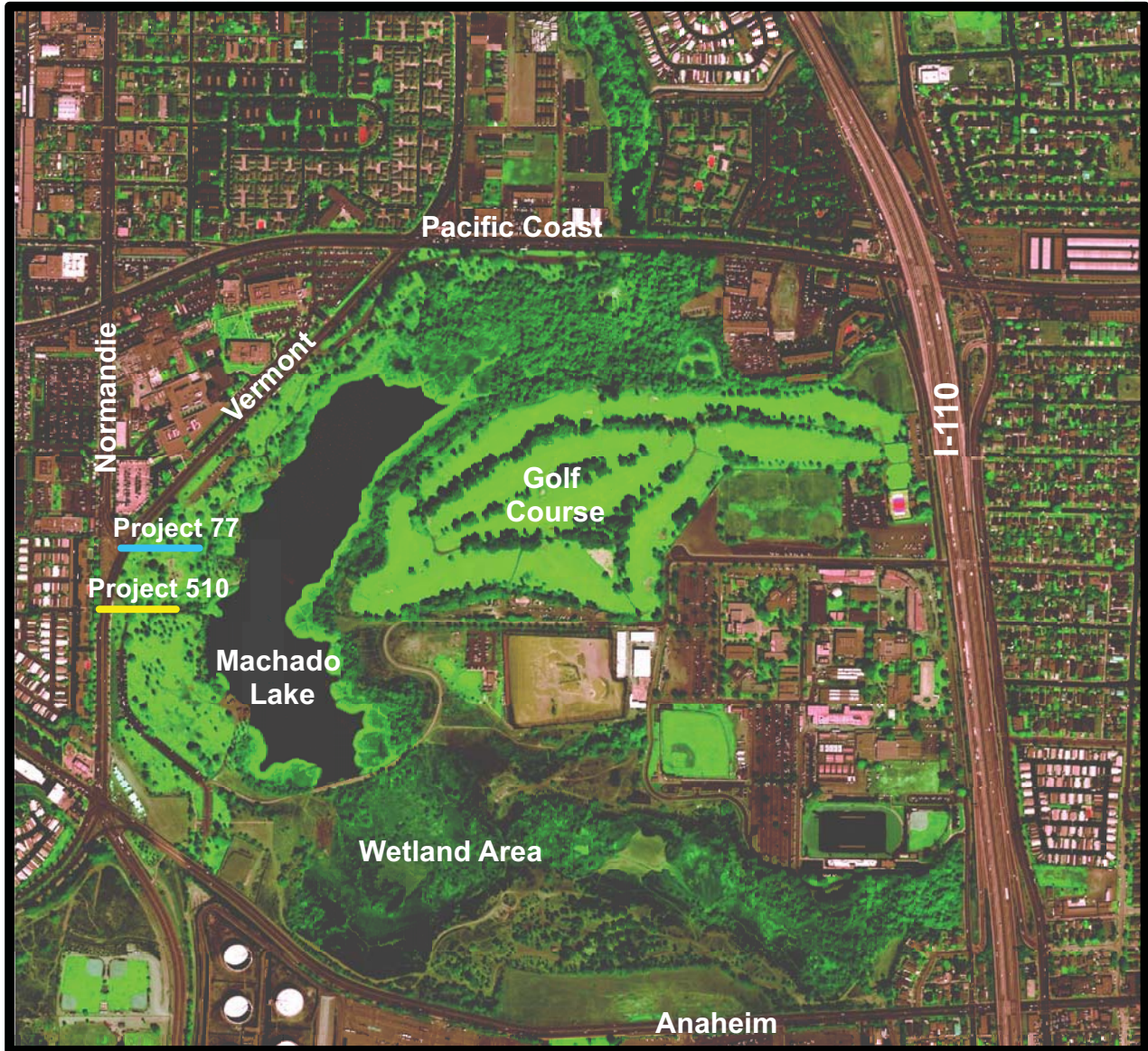
Figure 4 2007 Satellite Imagery of Machado Lake and Ken Malloy Harbor Park Overview
