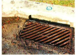
**Figure 3.** UltraDrainguard-protected inlet showing water flow bypassing the filter and entering the curb opening.
