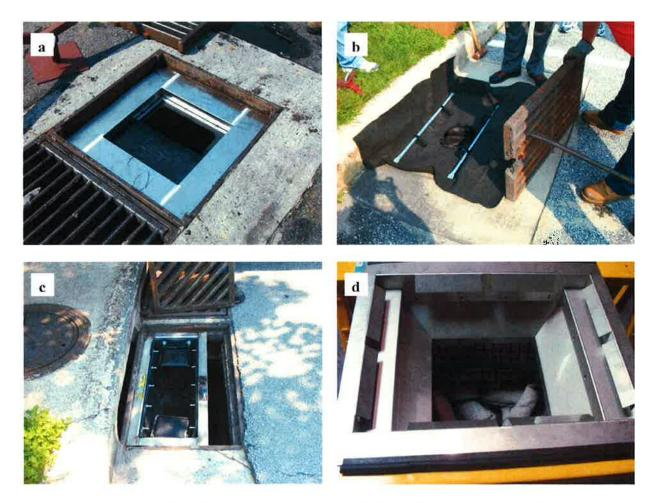
**Figure 1.** Photographs of installed catch basin inserts. (a) HydroKleen units at the I-95 service plaza; (b) UltraDrainguard filters at the service plaza; (c) DrainPac inserts in Drummond North subdivision; (d) FloGard Plus units at the Wilmington Riverfront.
