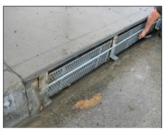
Figure 1.4 Automated Retractable Screens
