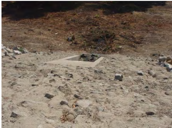
1. View looking down at outfall
