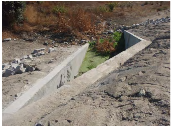
2. View from above outfall
