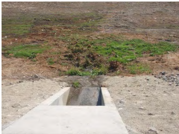
3. View looking down at outfall
