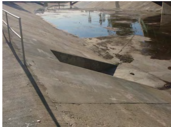
2. View of outfall
