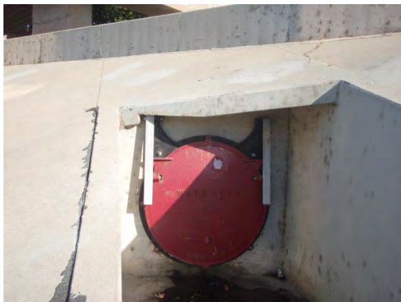
3. View of outfall
