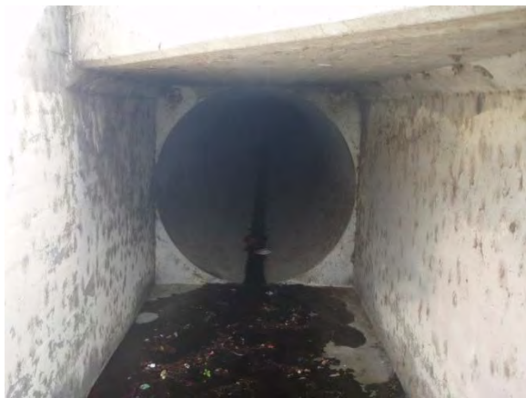
3. View of outfall
