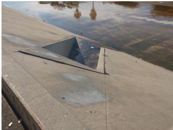
1. View of outfall from bike path
