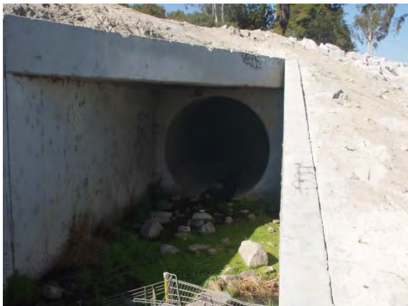
3. View of outfall
