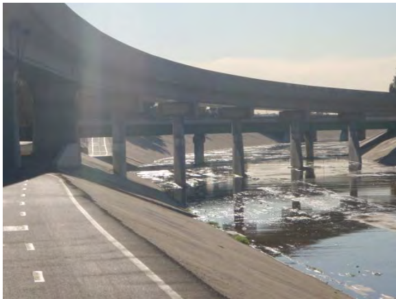
1. View of outfall north of railroad bridge
