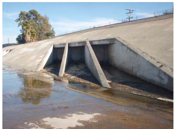
4. View of outfalls from Rio Hondo
