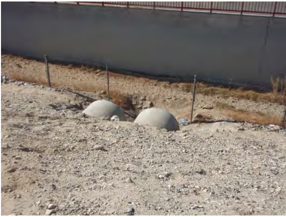
5. Possible inlets on west side of bike path
