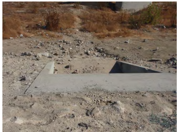
2. View from above outfall
