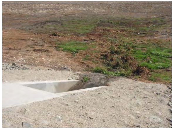
2. View looking down at outfall
