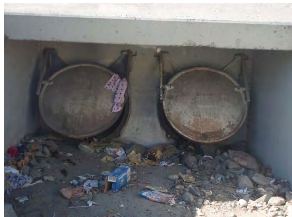
4. View of outfalls
