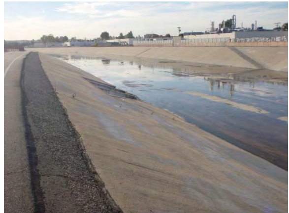
2. View looking South toward the three outfalls
