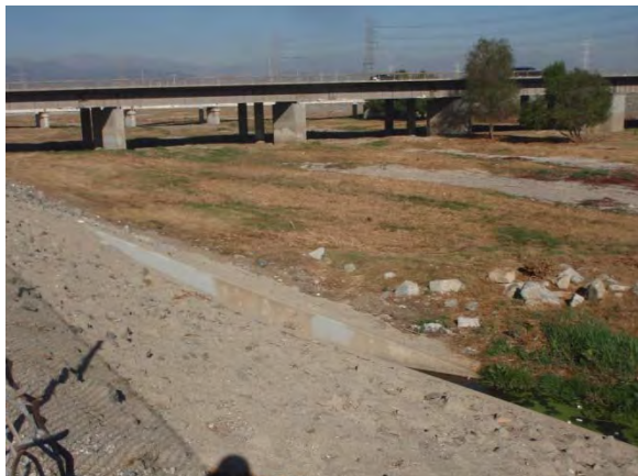
3. View of outfall looking towards Valley Blvd
