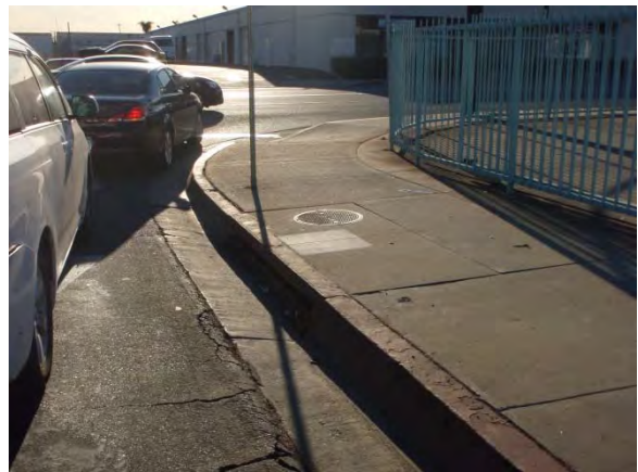
4. View of west catch basin
