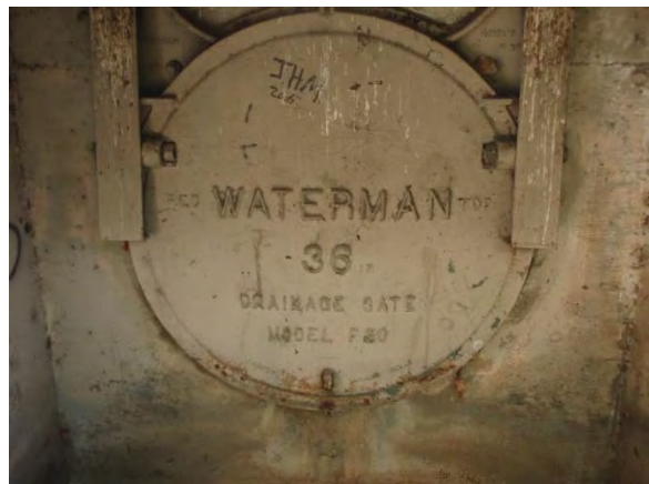
4. Close up of outfall
