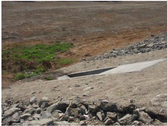
1. View looking down at outfall
