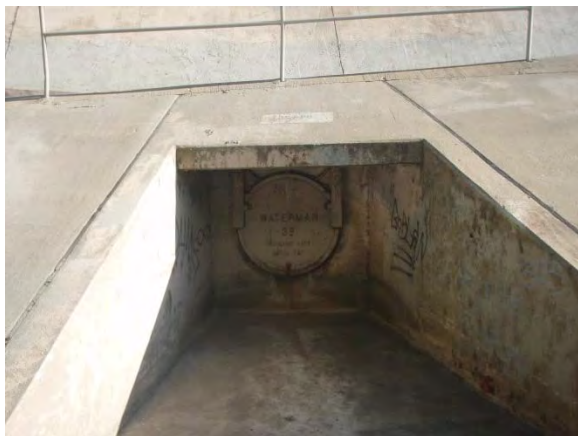
3. View of outfall
