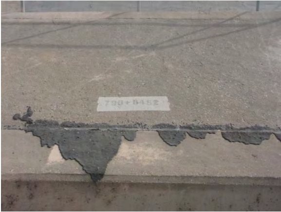
5. Markings near outfall
