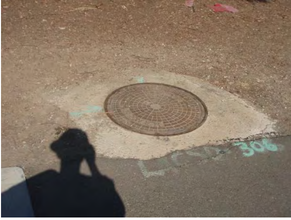
5. West manhole close up
