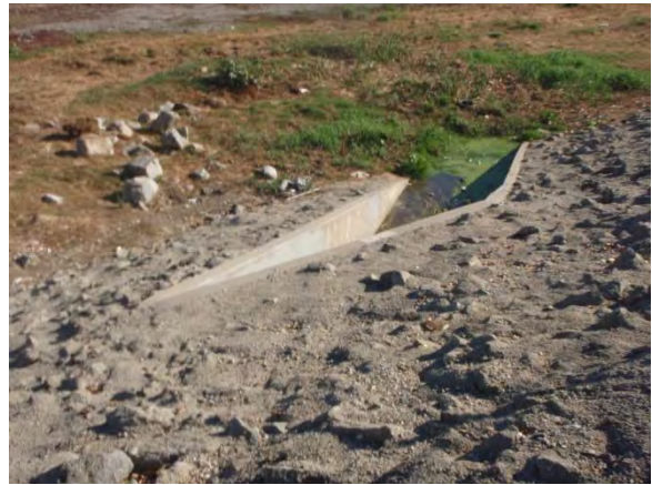
2. View from top of outfall
