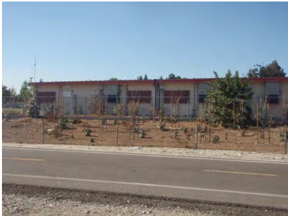
1. View across bike path opposite outfall
