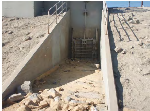
2. Close up view outfall
