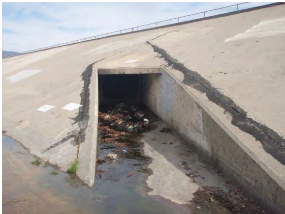
1. View of outfall from Rio Hondo
