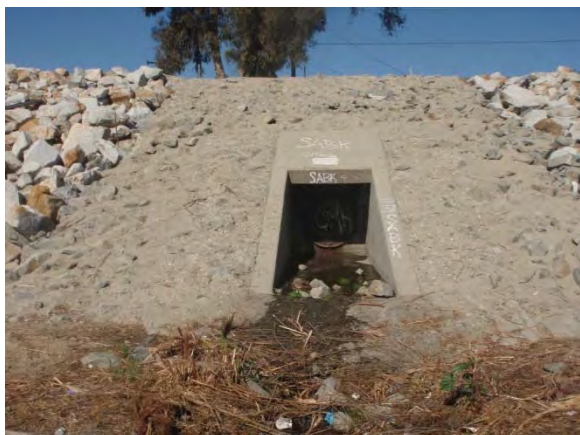
3. View of outfall
