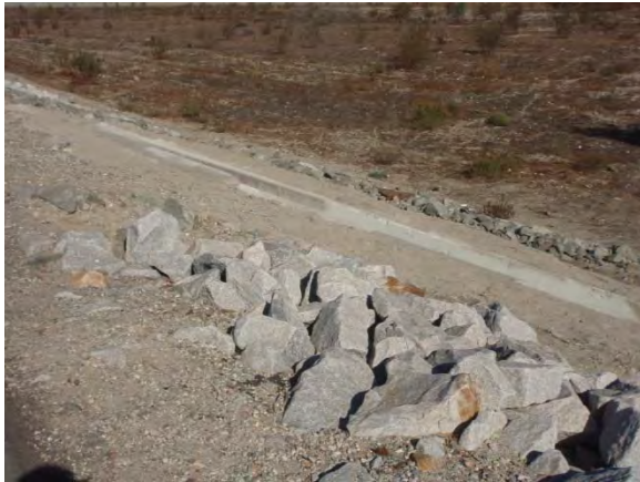
1. View looking down at outfall
