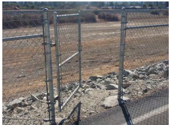
4. 5. Gate entrance near outfall
