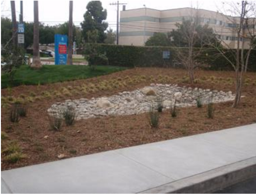
Figure 10: Infiltration Basin
