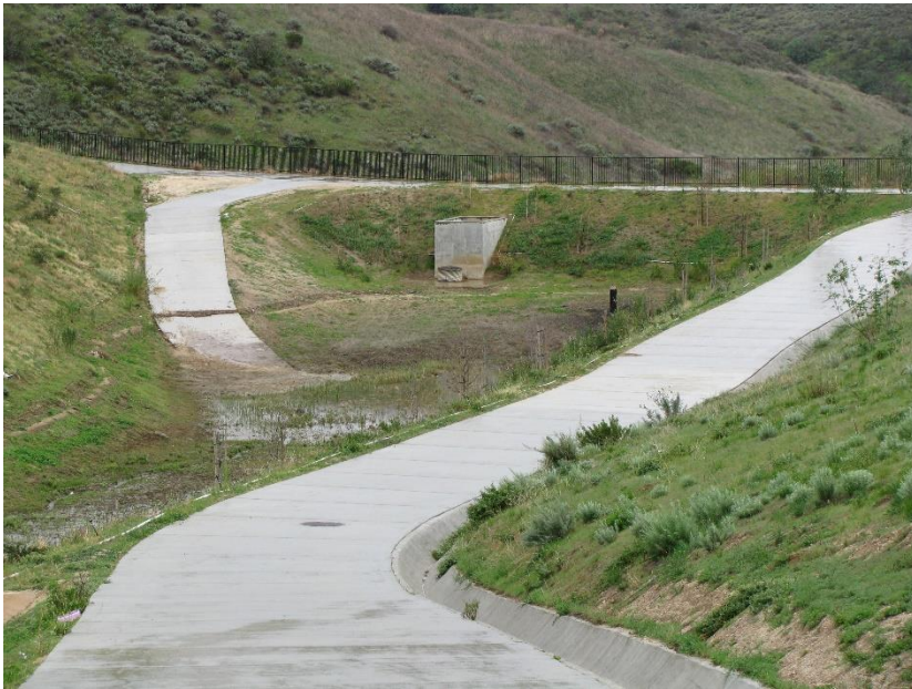
Figure 11: Extended Detention Basin
