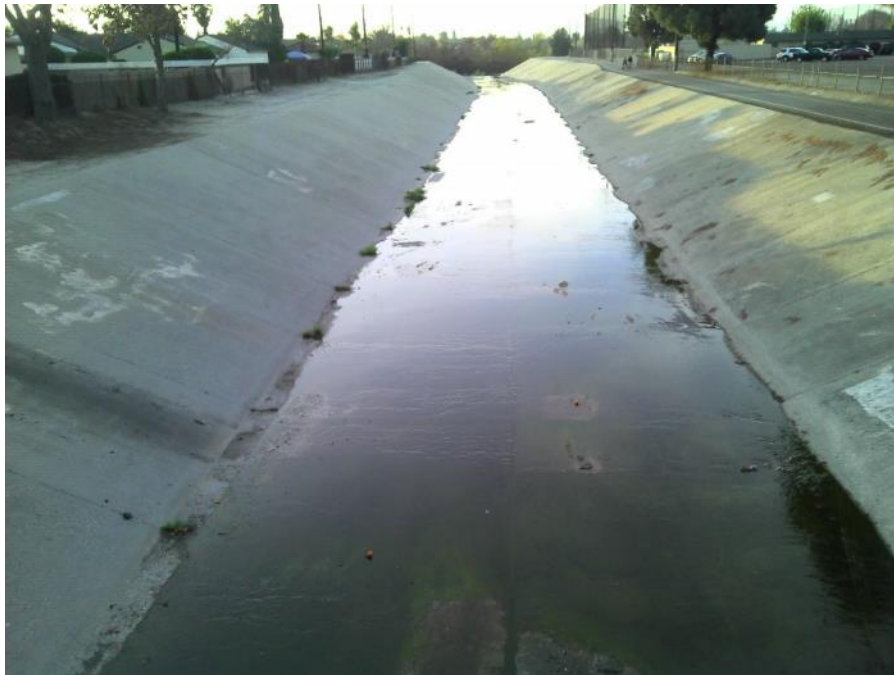
RHSGR_SAN_DD Looking Downstream
