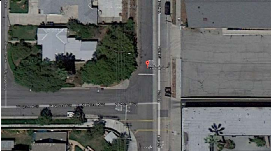
BI 0025 Peck Road Drain Aerial View
