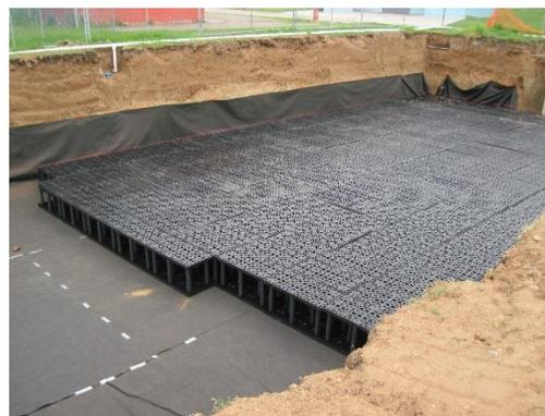
**Figure 5-5. Subsurface infiltration gallery being constructed below a public park (source: Tetra Tech)**
