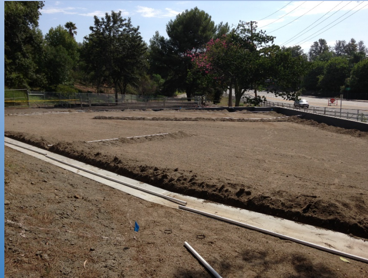
Construction of Biofiltration System
