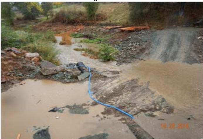
Photo 9. Sediment flowing downstream as a result of the dam breach. Note lack of BMPs around the work site.
