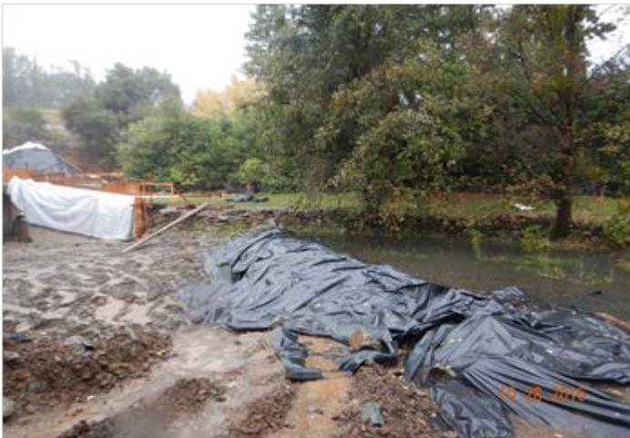
Photo 7. View of the plastic-covered diversion dam. Note: the area where water is seeping under or through the dam.
