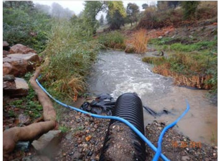
Photo 2. Clean water discharging downstream of the bridge project. Note: blue hoses used to dewater the construction area.
