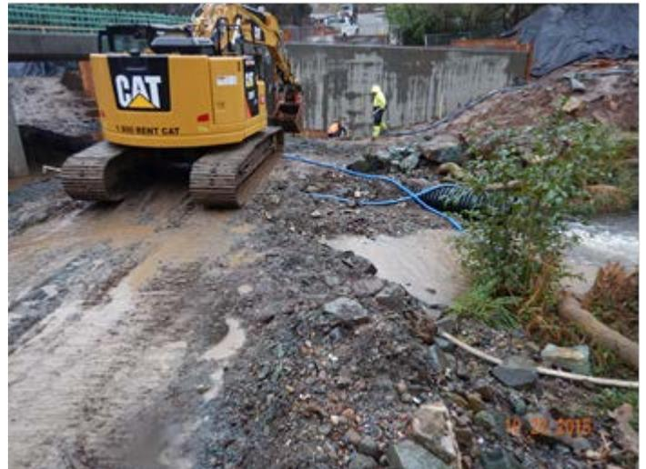
Photo 4. View of the work area early in the inspection. The work area had an earthen surface without BMPs.
