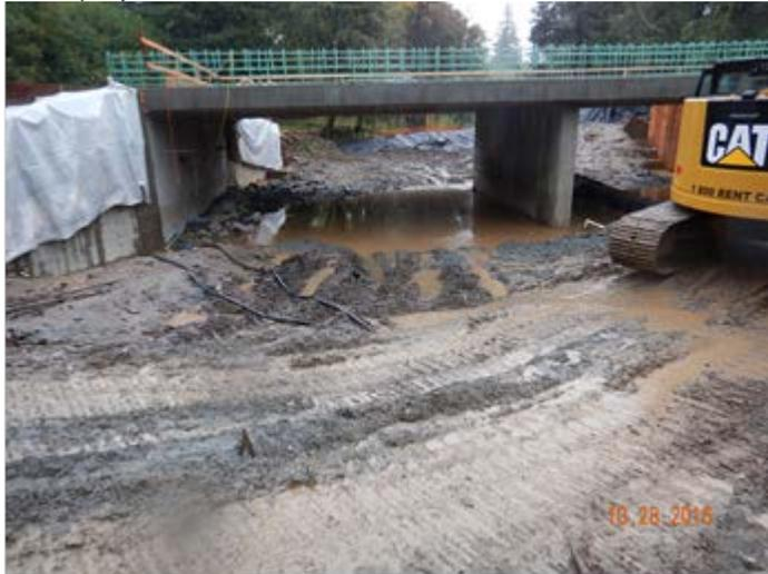
Photo 3. View of work area looking upstream. Note lack of storm water BMPs
