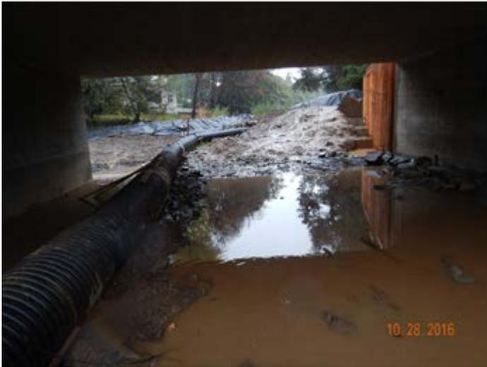
Photo 1. View of area under new bridge looking upstream. Black diversion pipe extended under bridge and through the project.
