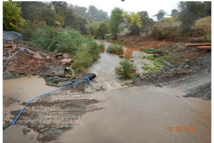
Photo 10. Another view of the downstream storm water discharge. Note: the turbid storm water discharging downstream.
