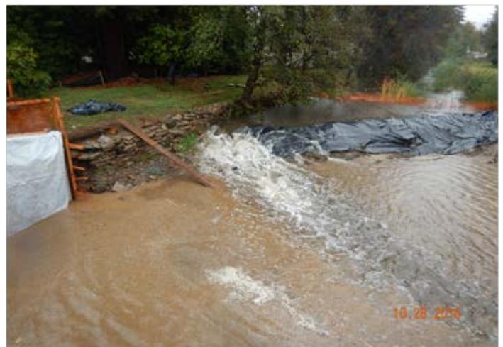
Photo 10. View of creek flow overtopping dam with significant amount of water flowing into the work area
