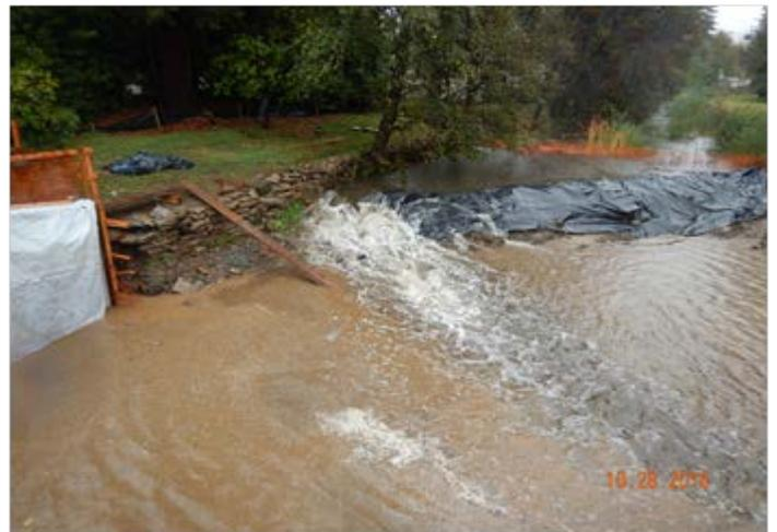
Photo 10. View of creek flow overtopping dam with significant amount of water flowing into the work area
