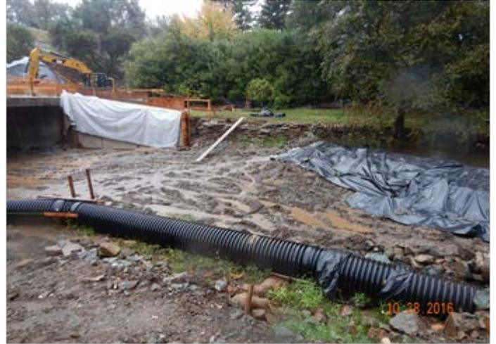
Photo 8. View of diversion dam as water was starting to overtop north end.
