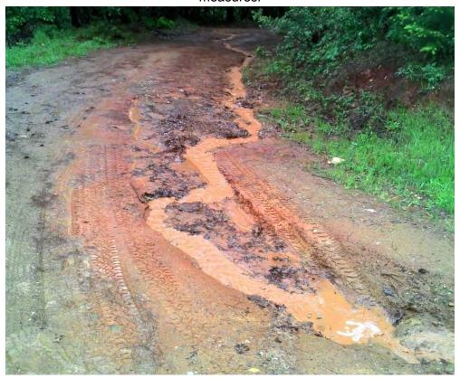
Photo 5. Main Access Road exhibiting heavy sheet flow, erosional scarring, and lack of erosion control measures.
