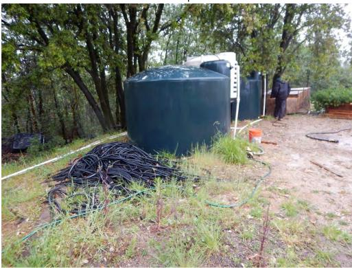
Photo 26: Irrigation pipes from the storage tanks. Weathered staked straw waddles installed behind the water tanks—providing little protection from runoff and erosion.
