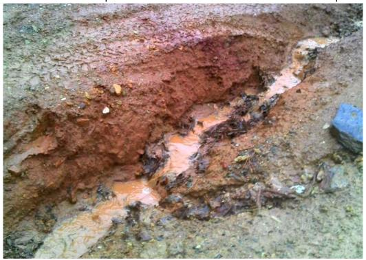
Photo 10. View east: turbid sheet flow exiting road into forested drainage. Way Point 087.
