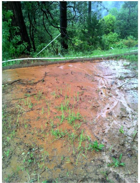
Photo 3. Straw waddling installed for sediment control.
