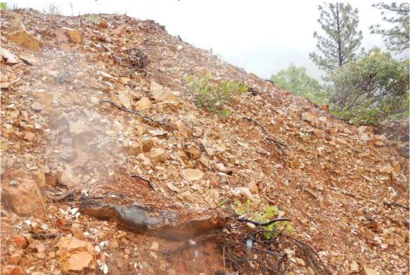
Photo 56: Unprotected cut-slope from bottom terrace to second terrace.
