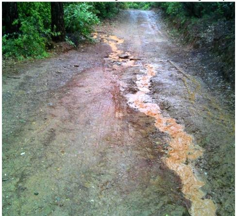
Photo 11. Turbid sheet flow exiting road into forested drainage through ineffective slash. Way Point 087.
