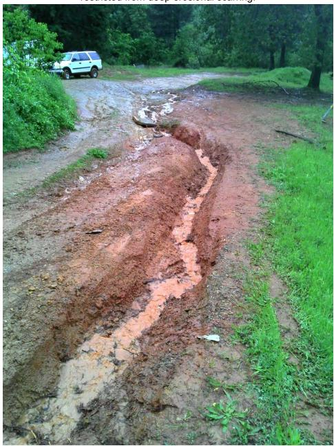
Photo 9. View East – Close-up view of extensive erosion on Main Access Road up to the Site.
