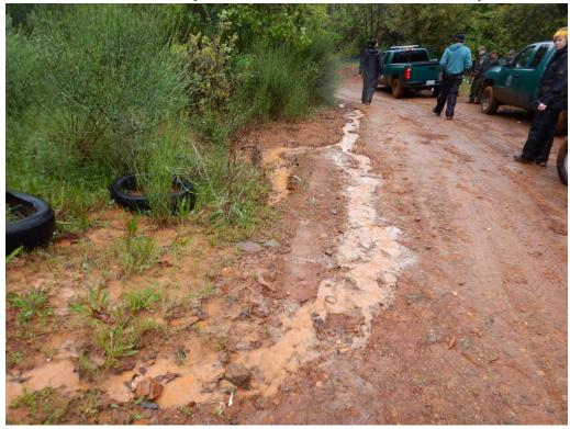
Photo 17. Looking northeast, turbid runoff exits road and property flowing towards Canyon Creek. Way Point 089.
