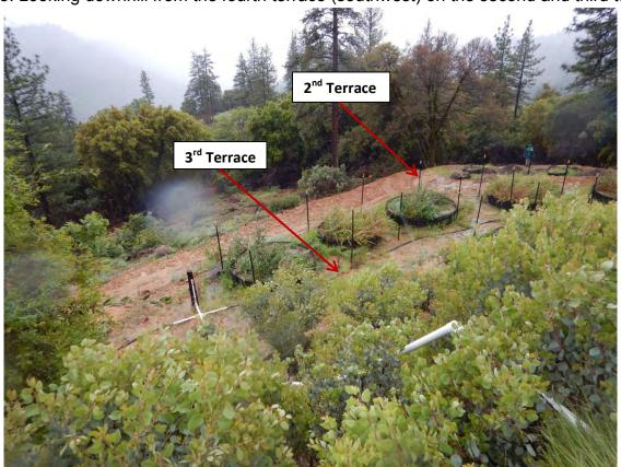
Photo 54: Bottom terrace. Note "sediment trap: to the left and slash to the background.
