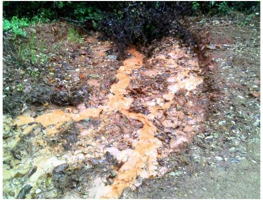
Photo 12. Turbid sheet flow exiting road into forested drainage through ineffective slash. Way Point 087.
