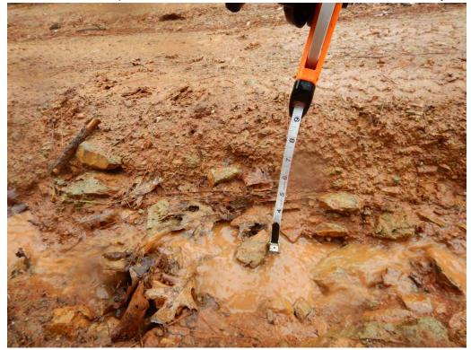
Photo 8. View North East - Extensive erosion on Main Access Road up to the Site. Vehicle access severely restricted from deep erosional scarring.
