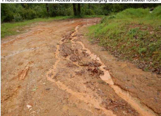
Photo 6. Erosion on Main Access Road discharging turbid storm water runoff.
