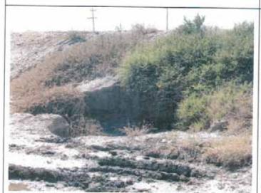
Photo 2: Large hole on the eastern embankment of the 'Big Reservoir.' It appeared to staff this hole compromises berm integrity.
