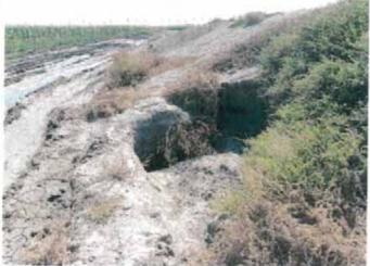
Photo 3: Large hole on the eastern embankment of the 'Big Reservoir.'
