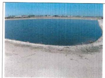
Photo 1: Typical condition of all storage lagoons at the facility. No signs of berm erosion and/or animal burrowing. Note 3'-5' freeboard.
