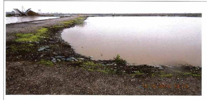
Photo 4: Photo of the lagoons onsite at capacity without the required freeboard.
