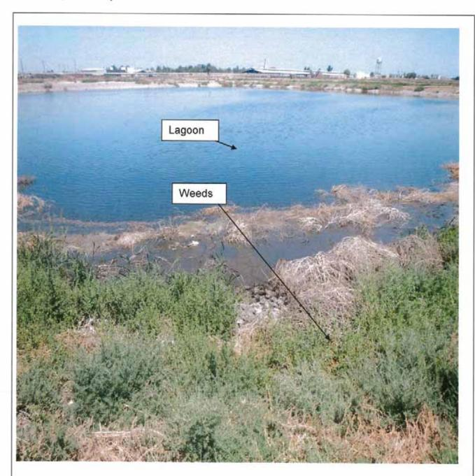
Photo 5: Photo of a lagoon with excessive vegetation on its inner and outer embankments.
