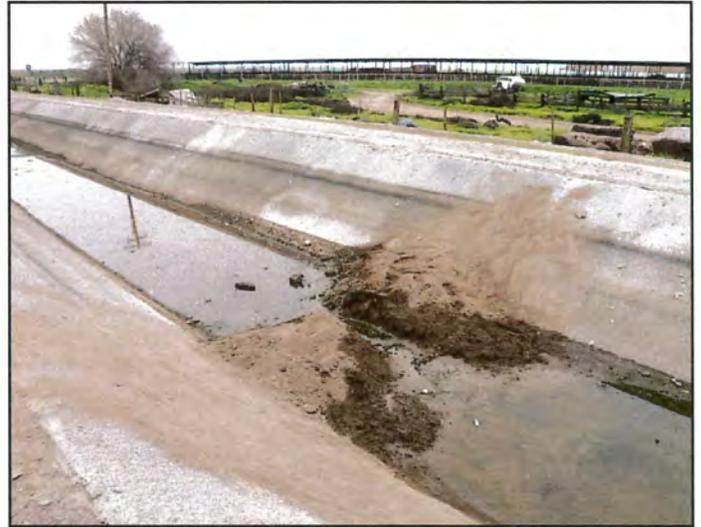
**01 22 2015** – View southeast showing berm in MID canal; note breach in center of berm.
