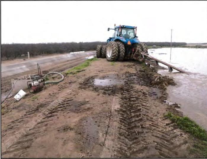
View east down north berm of Lagoon 2 showing pump intake at right and point of discharge at left; note lack of freeboard.
