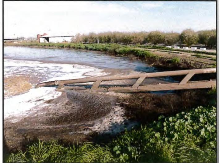
**02 26 2015** – View northwest across east end of Lagoon #1; note lack of freeboard. The pipe is part of the pumping mechanism for applying wastewater to cropland.
