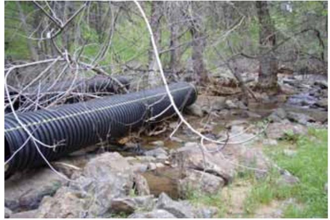
**Figure 10:** Culverts which washed down stream from the dam failure area
