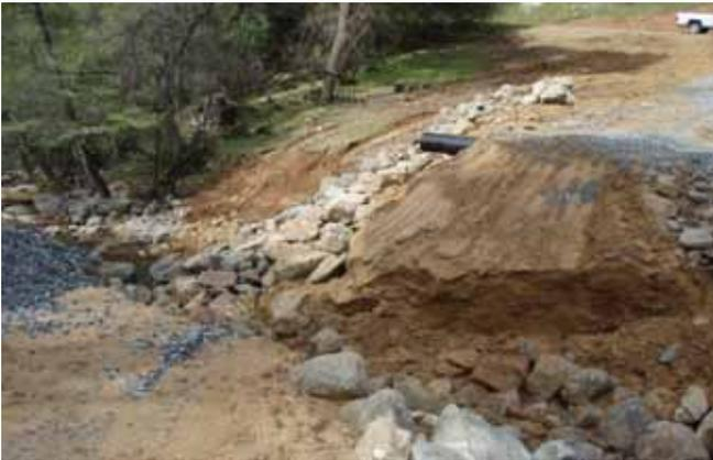
**Figure 3:** Area where the earthen dam failed
