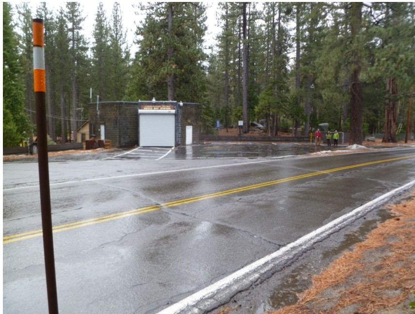
Figure 1-11. Meeks Bay Fire Station when viewed from across Hwy 89. The structure is extremely small and does not meet the needs of the fire crew stationed there.
