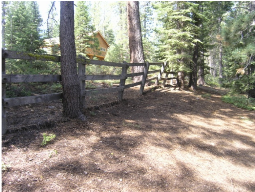
Figure 1-5. Evidence of sheet flow (water flowing evenly over a surface) from the subdivision onto the William Kent campground site (point B on the map in Figure 4).
