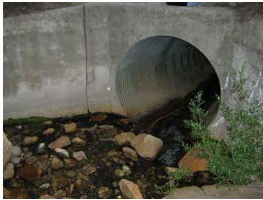
Culvert below sampling site at Little Cottonwood Creek (7/13/11)
