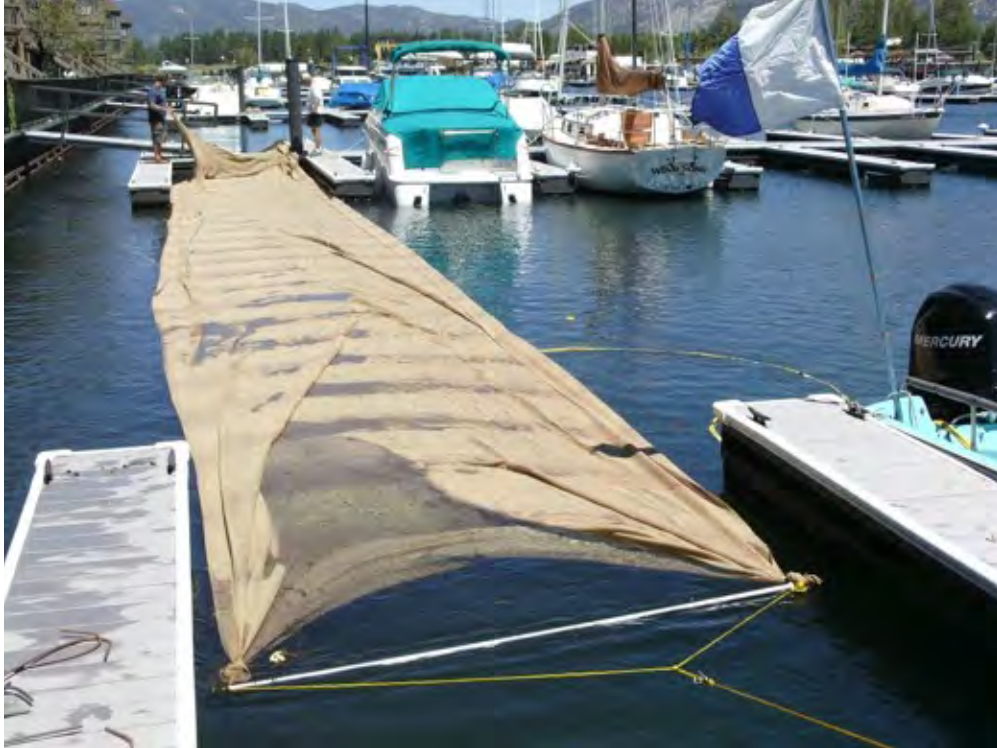
Figure 10. Jute Bottom Barrier
