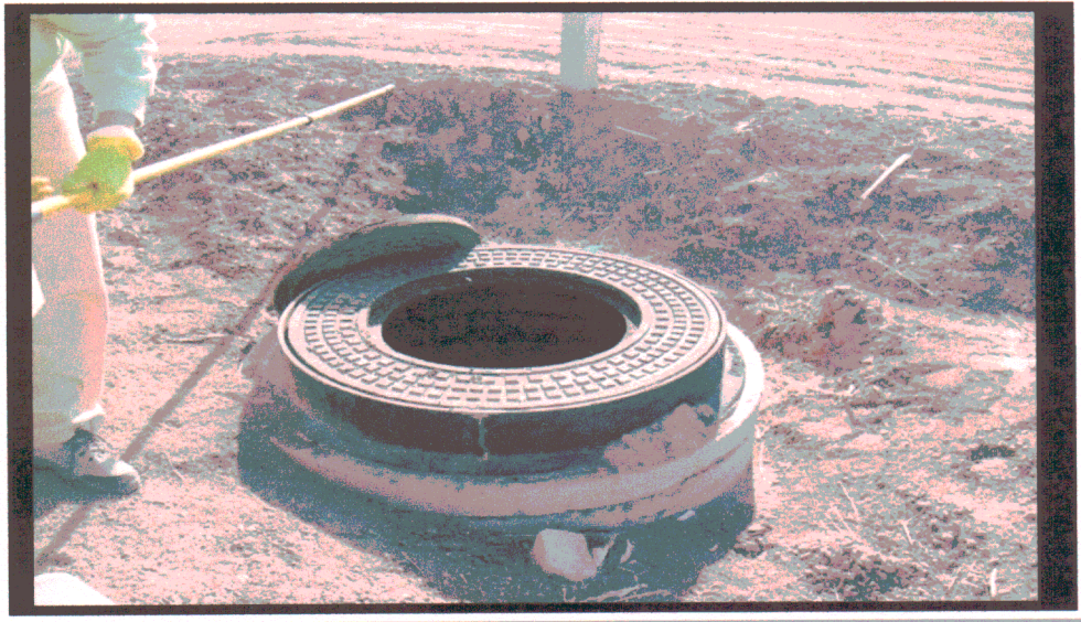
Sample taken at Discharge Manhole Access Central Drain 3D No 1 (undergrounded)
