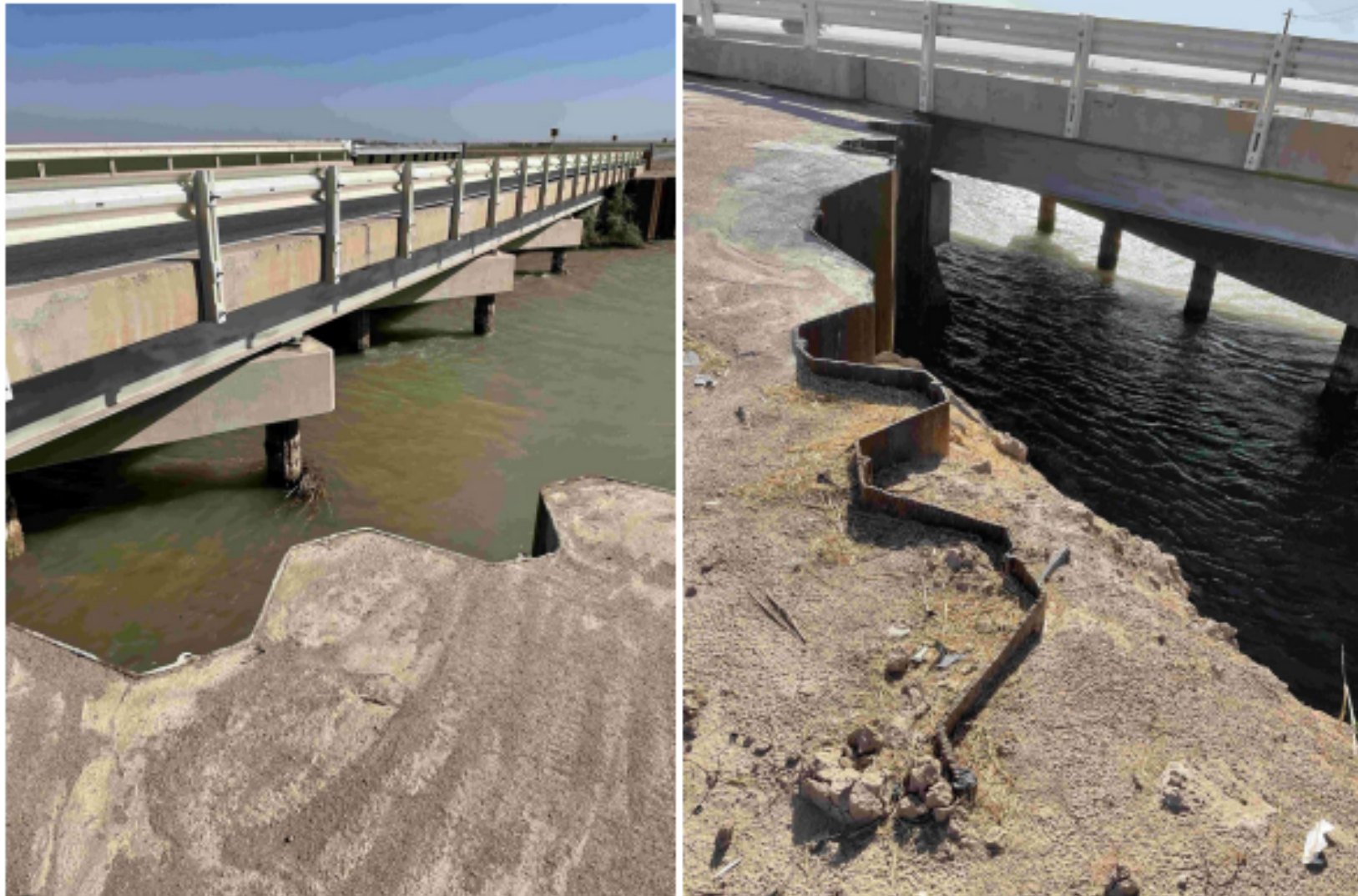
Figure 4: Photos of the existing Forrester Road Bridge and Westside Main Canal.
