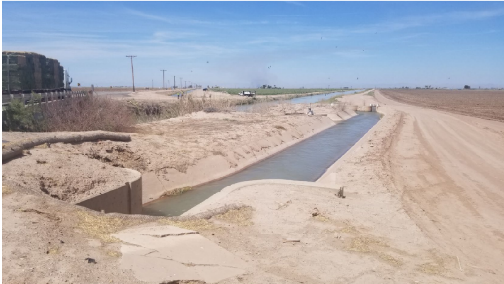
Figure 5: Photo of the existing Sumac Lateral Canal.
