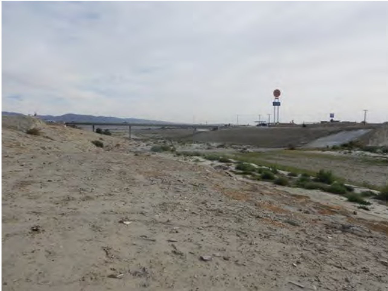
Photograph 3: View of the Whitewater River/ CVSC Facing Southeast Towards the Monroe Street Overcrossing
