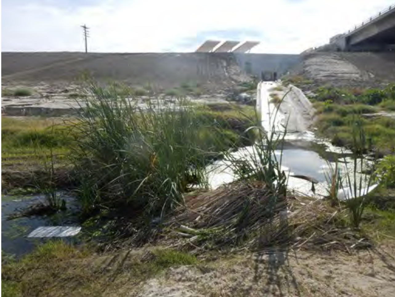
Photograph 4: View Facing South Depicting Drainage 2
