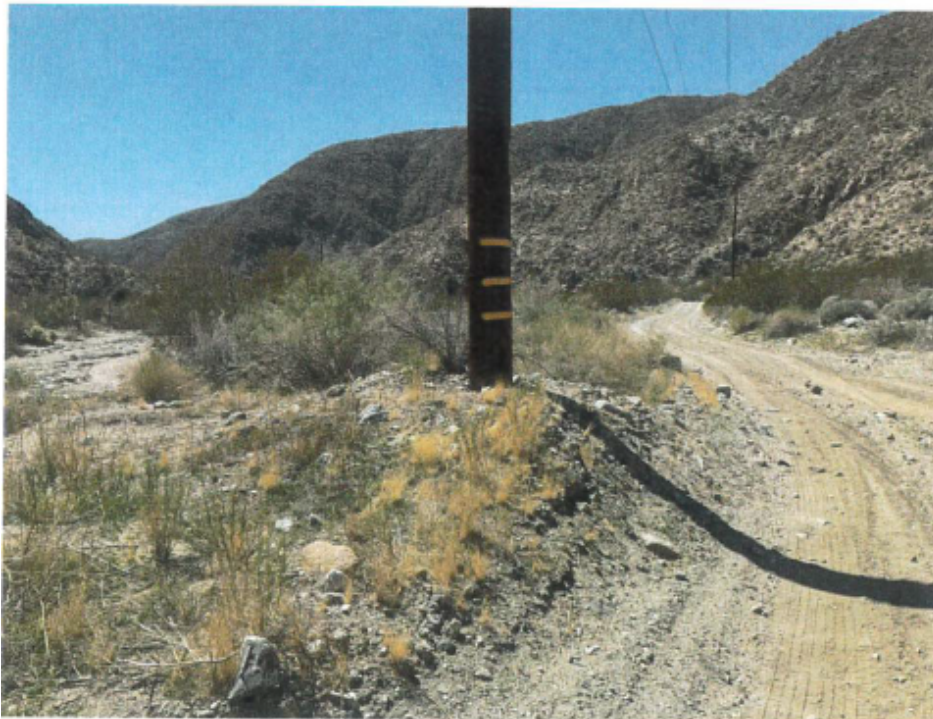
Photograph 4: Pole A13721186E Base. Photo Facing Southwest (Downstream)
