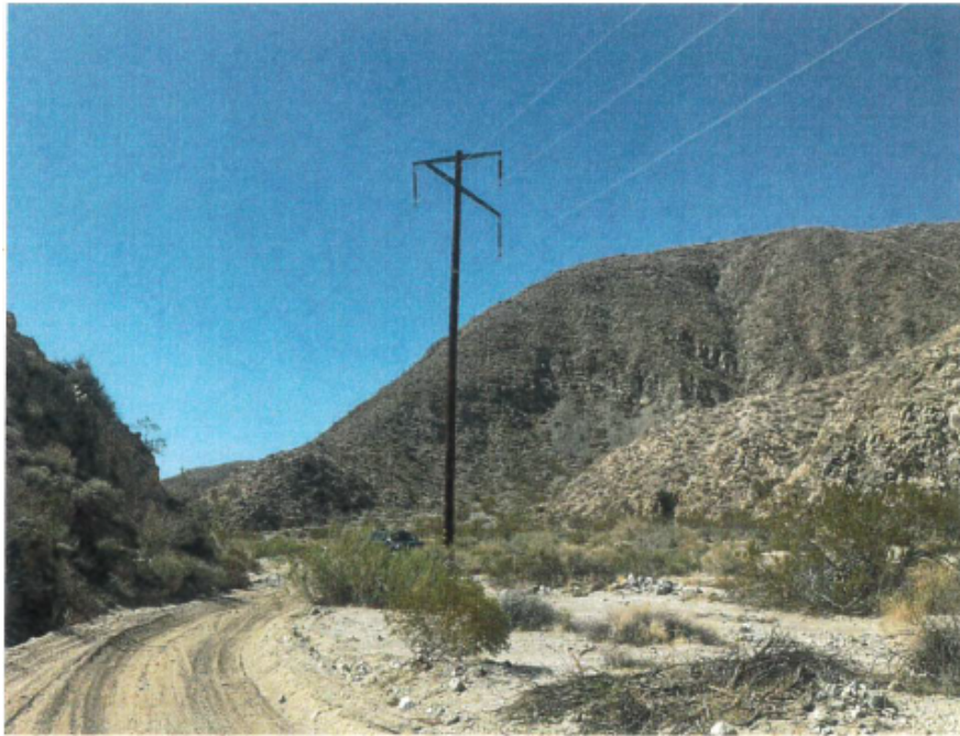
Photograph 3: Pole A13721183E Overview. Photo Facing South (Downstream)
