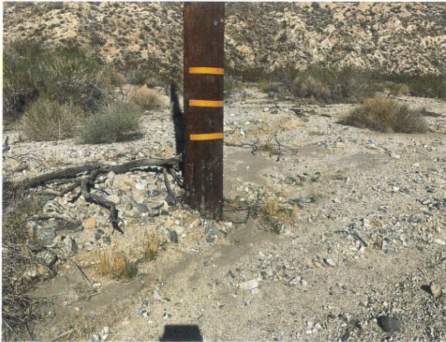
Photograph 1: Pole A13721182E Base. Photo Facing Northwest (Upstream)
