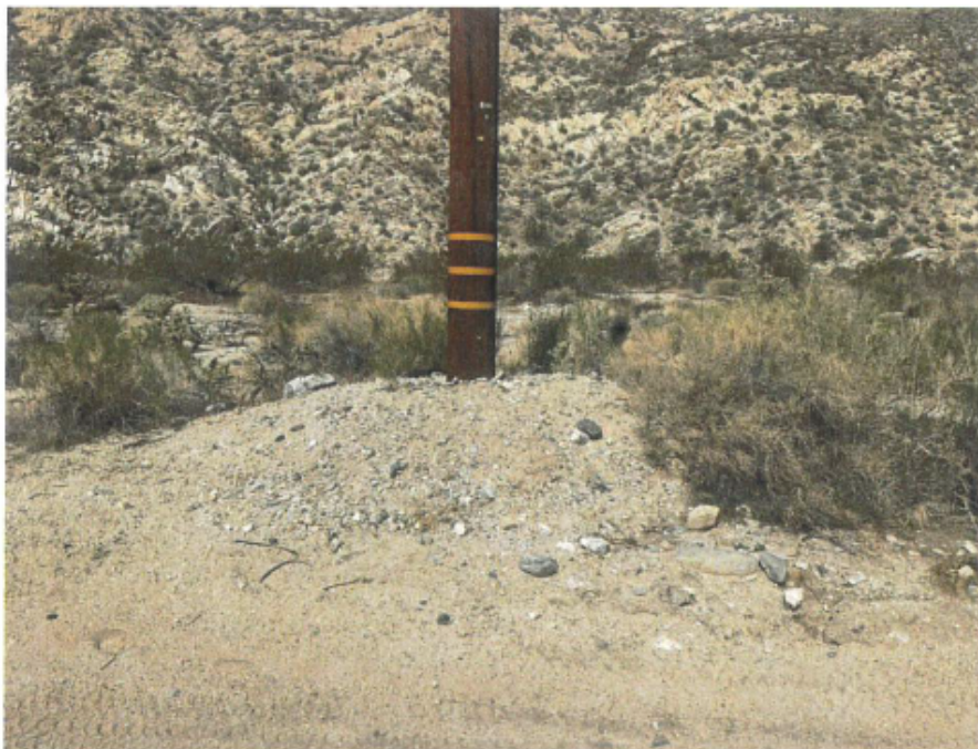
Photograph 4: Pole A13721183E Base. Photo Facing West (Downstream)
