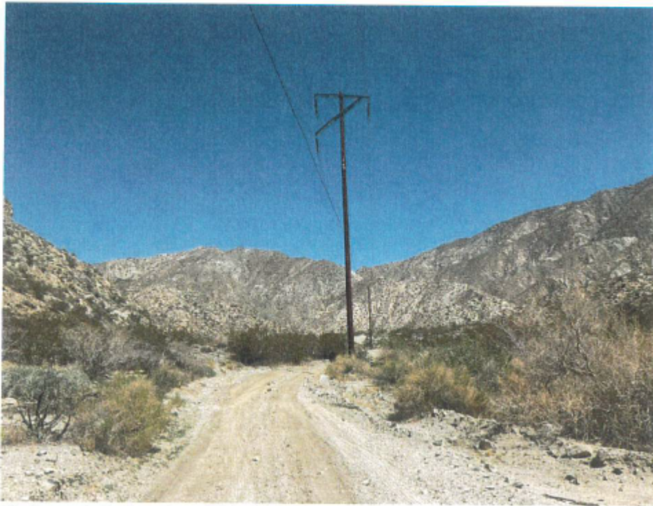
Photograph 3: Pole A13721186E Overview. Photo Facing Northeast (Upstream)
