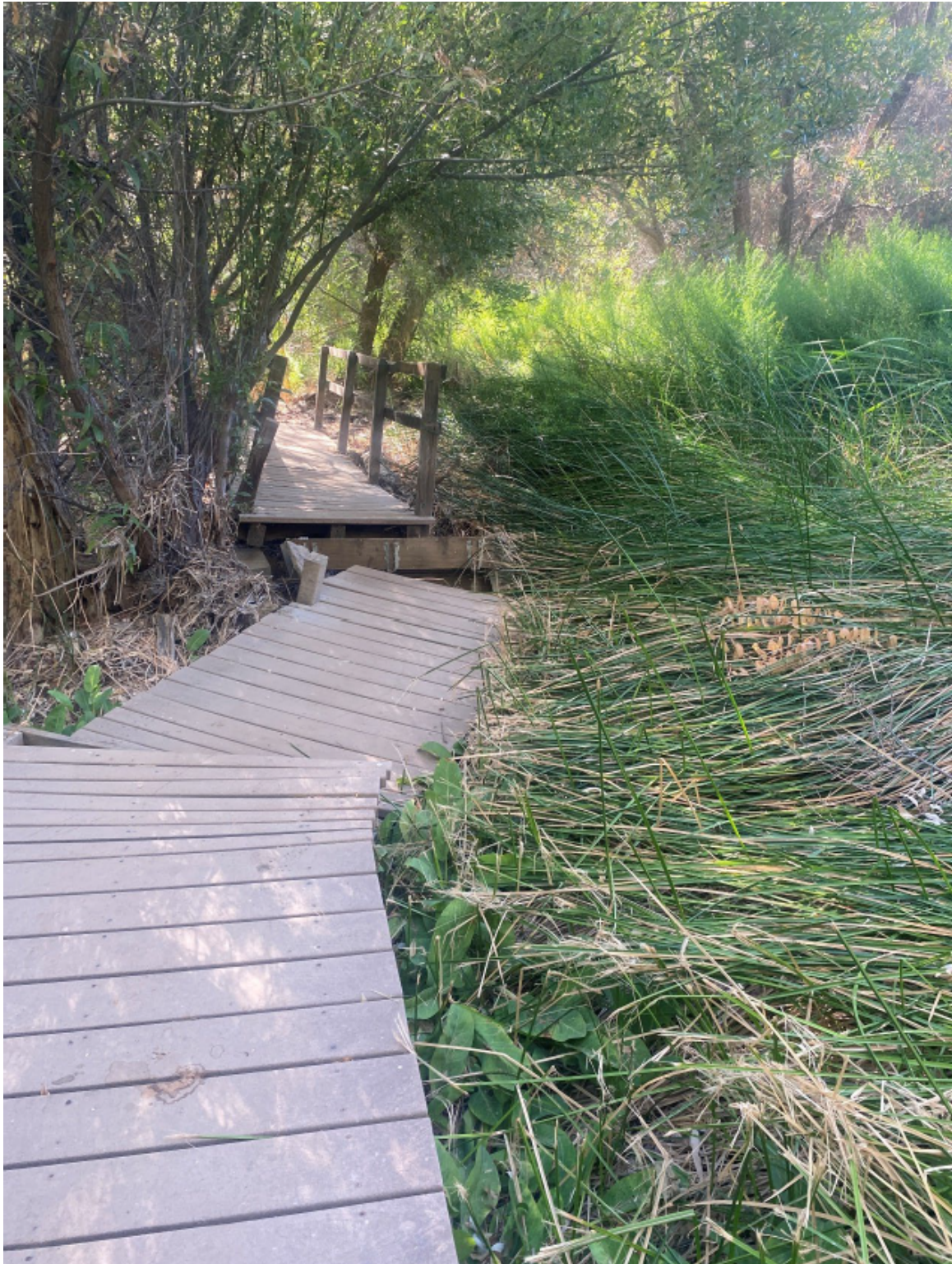
Figure 7. Photograph showing the boardwalk deck that will be replaced at Site 4 .
