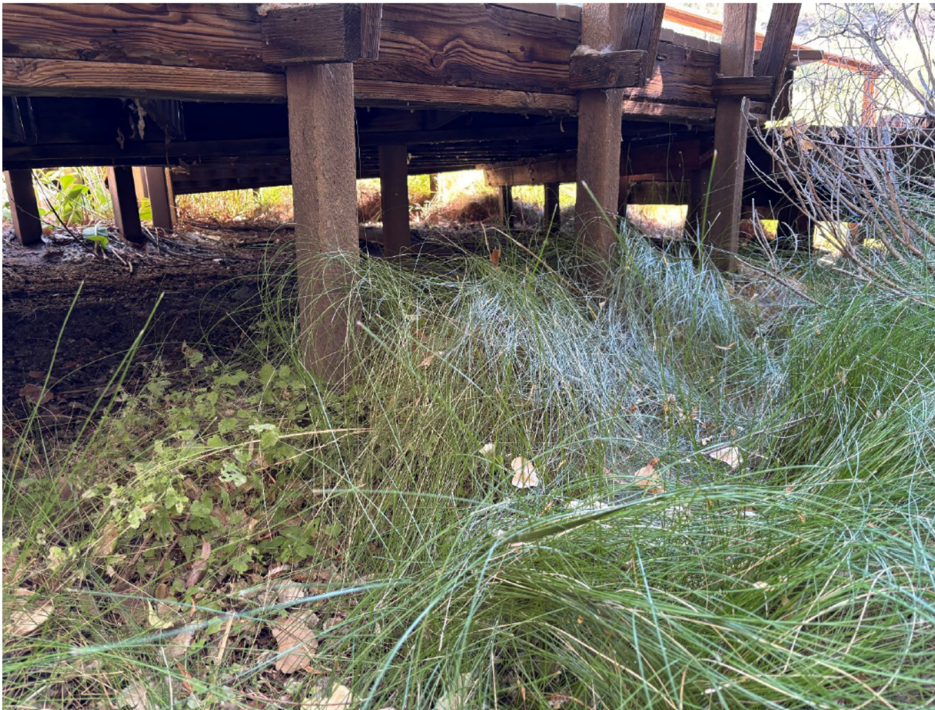
Figure 6. Photograph showing the boardwalk pilings that will be replaced at site 3.
