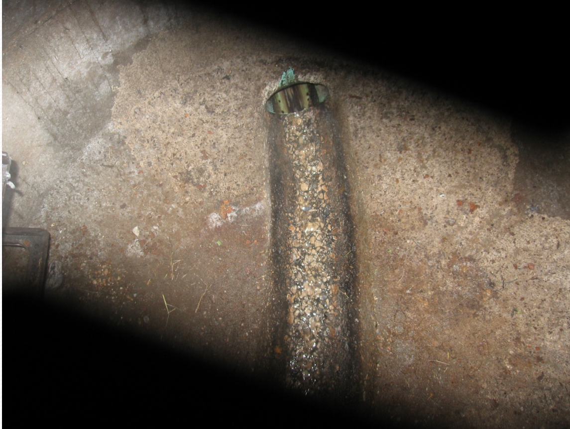
Sewer corrosion below a coffee shop
