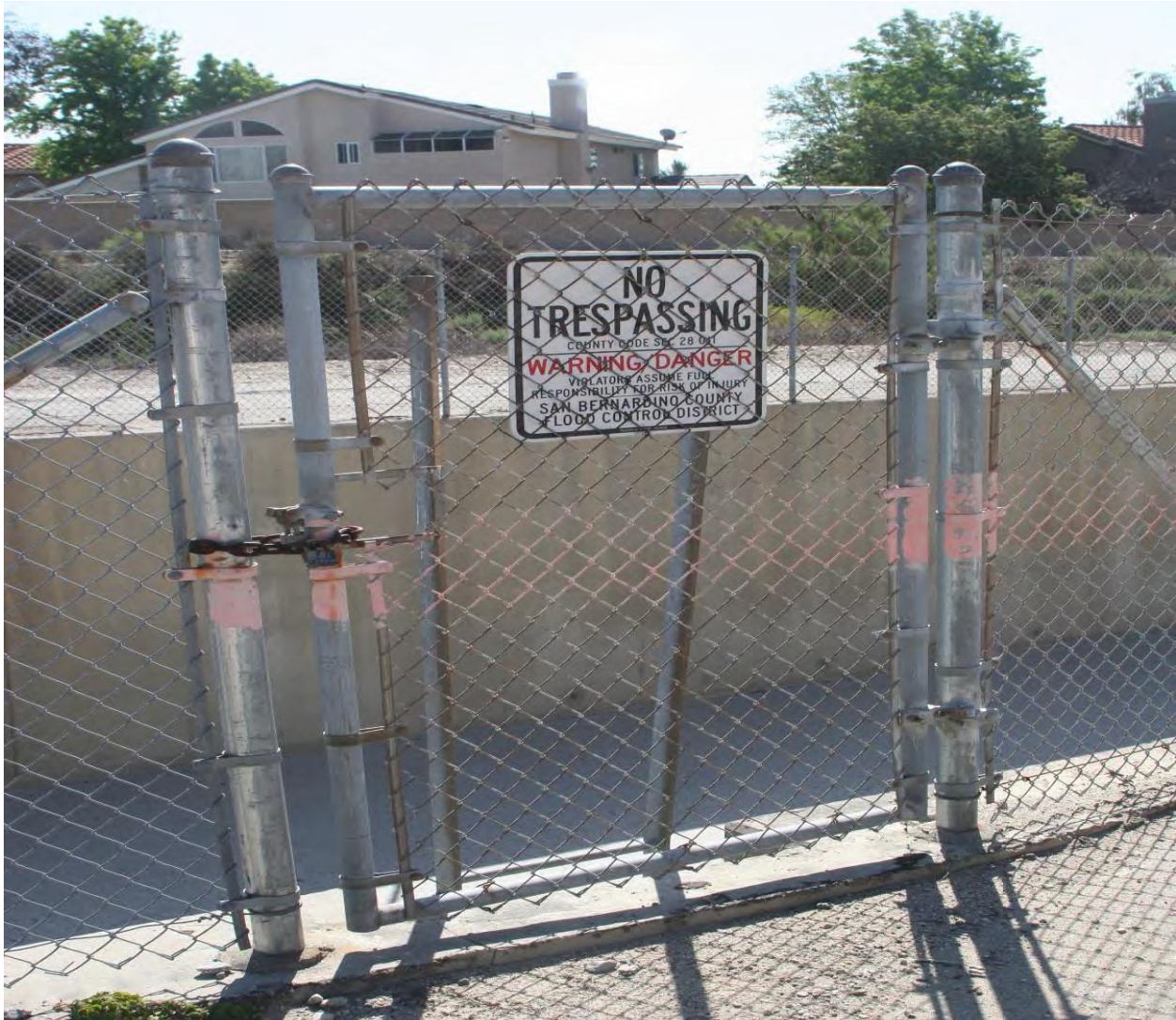
Figure CC-13. Reach 1, showing locked gate, fencing, and no trespassing/warning sign. The entire Reach is fenced with locked gates and posted to keep individuals out. All of the UAA waters are fenced and posted in a similar fashion to prohibit access.
