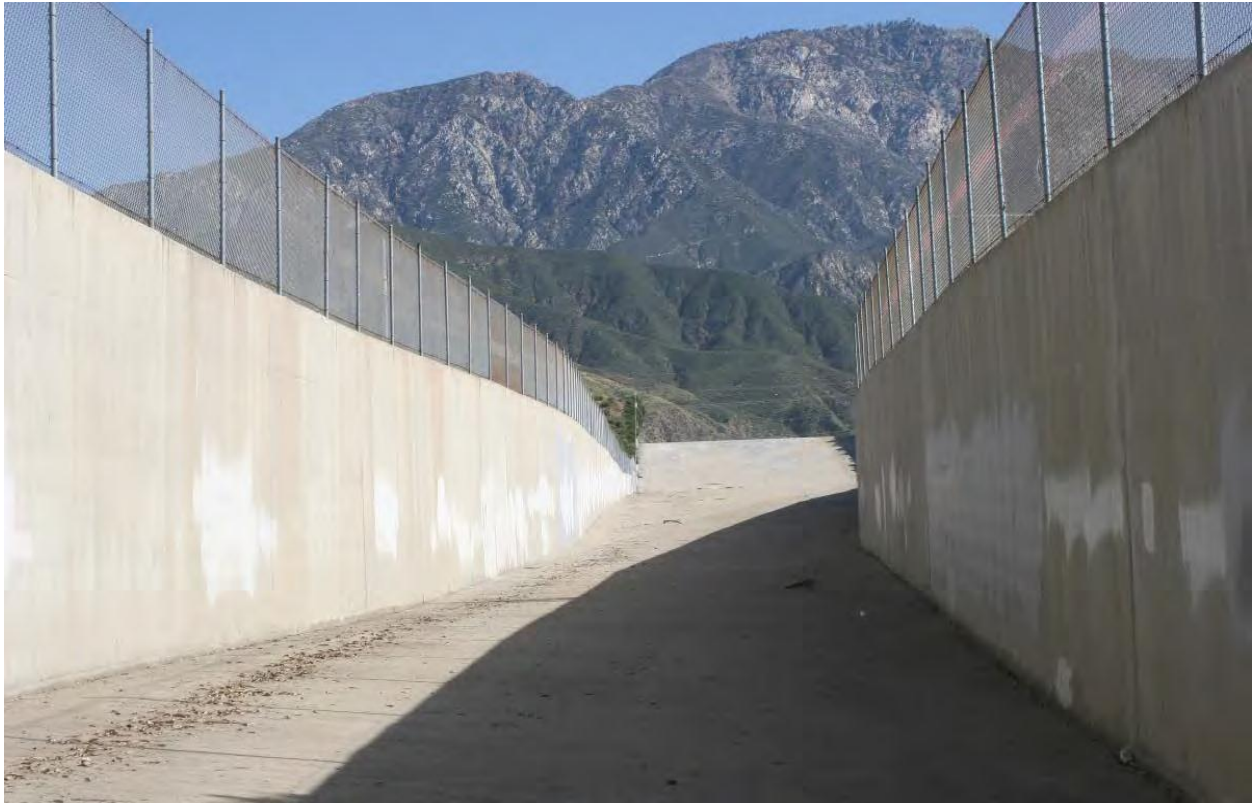
Figure CC-7. Reach 1, looking at upstream terminus (Cucamonga Canyon Dam) of Reach 1.
