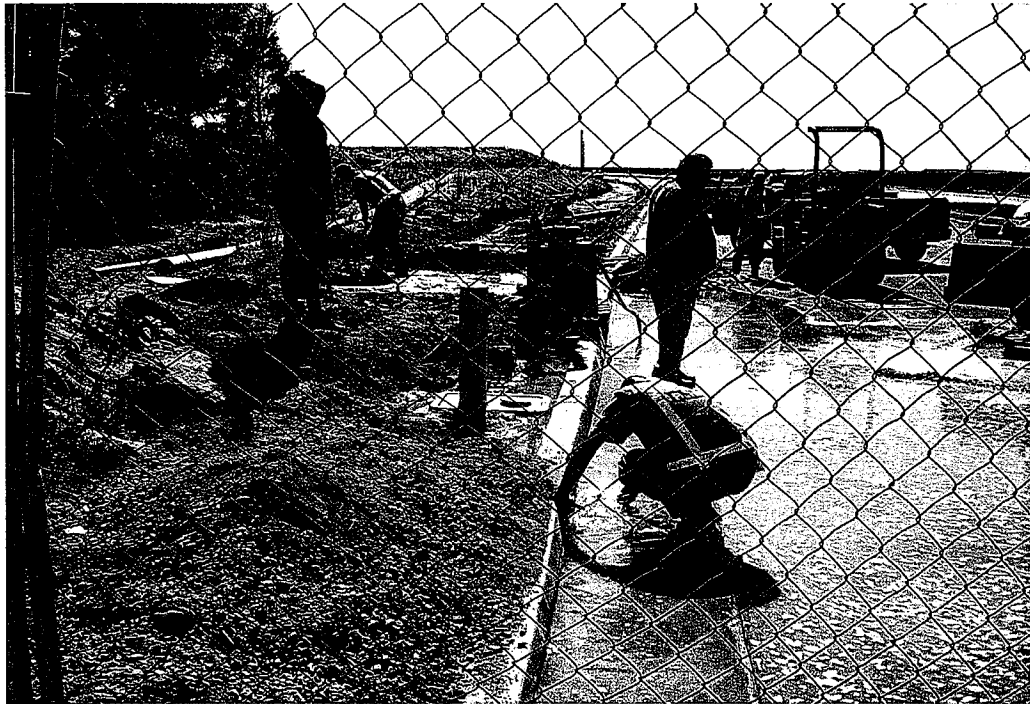
Photo 03: Workers attempting to shut off the water main. The SWPPP person, Mr. Henry Martinez, and his supervisor were present at the time of the incident.
