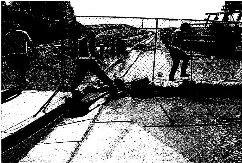
Photo 01: Ashby, USA workers attending to water line break. Initially, the workers were observed erroneously removing the gravel bags releasing the sediment-laden water along Murrieta Hot Springs Road.
