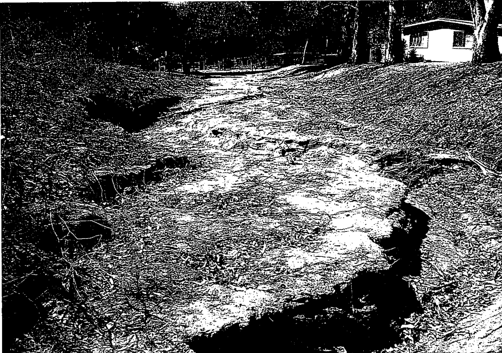
Photo 16: Complainant's property (5 acres) is to the left. Scouring of the embankment from erosion from low drainage flows. Per the complainant, during the wet season the erosion effects and sediment deposits are more pronounced in this area.
