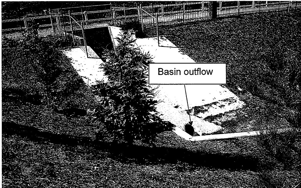
Photo 08: Placement of the basin outflow indicates the design is a flow-through system, eliminating settling time.
