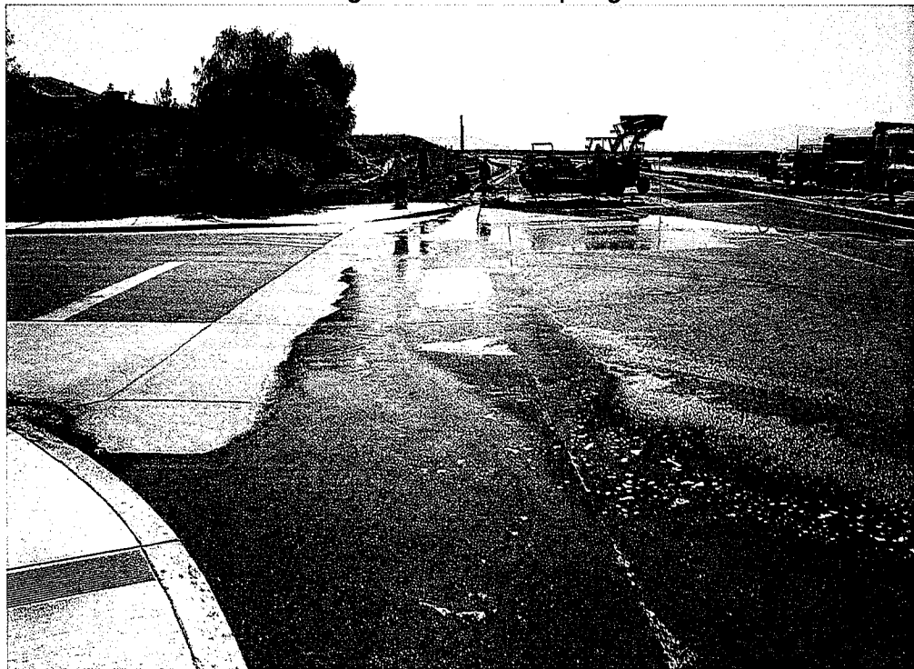
Photo 02: Our presence quickly alerted the Ashby works to maintain the BMPs, as sediment-laden water entered the storm drain along Murrieta Hot Springs Road.
