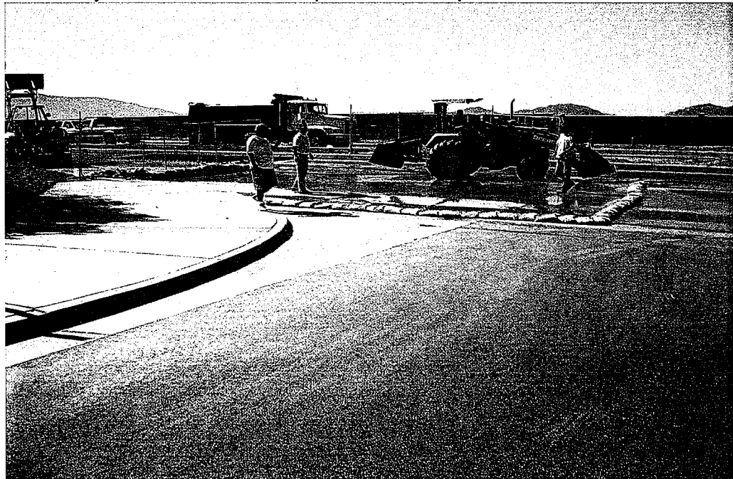
Photo 04: Sediment traps were immediately installed along Murrieta Hot Spring Road to contain and capture the sediment-laden water.
