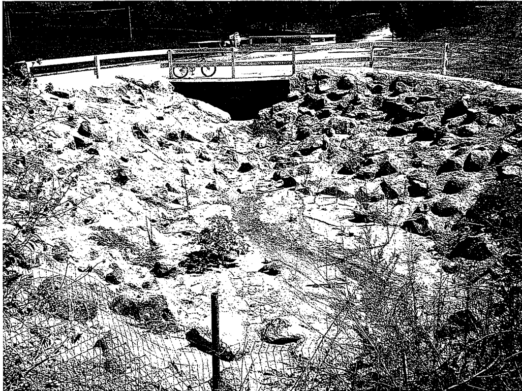
Photo 12: Culvert pipe-shows buildup of sediment deposit from discharges from sediment basin.
