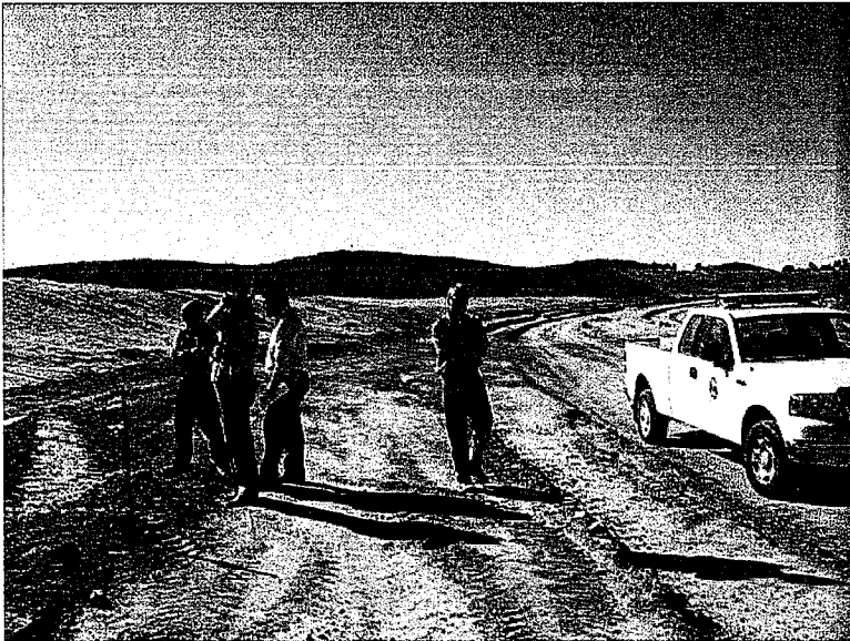
Photo 6. Loop Road bridge looking south. Additional BMPs are needed along road and at toe of slopes. Any unstabilized slopes should be stabilized.
