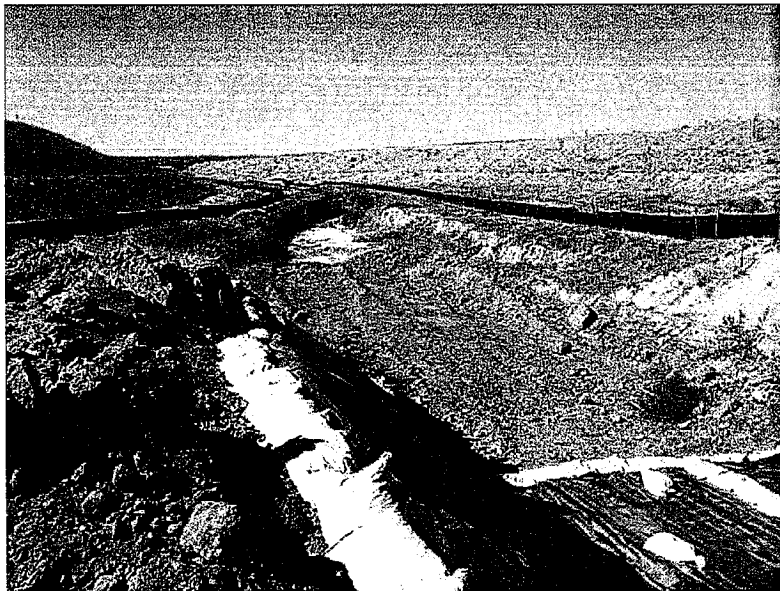
Photo 16. Long Valley Wash downstream of the berm in photo 15. Channel should be returned to its original state.
