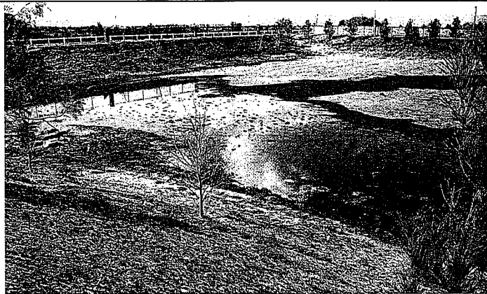
Photo 05: Looking northeast-extent of sediment basin with ponded water from runoff.
