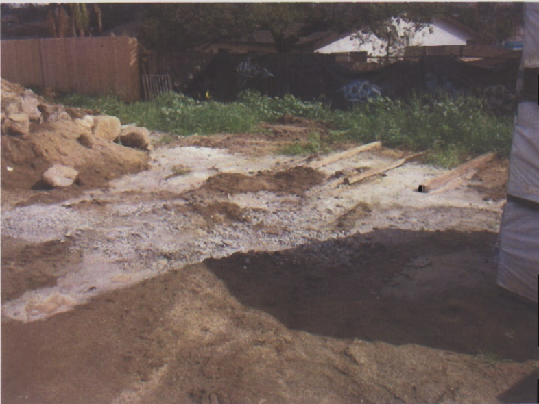
011. A concrete slurry spill on the ground. A washout was available across the street.
