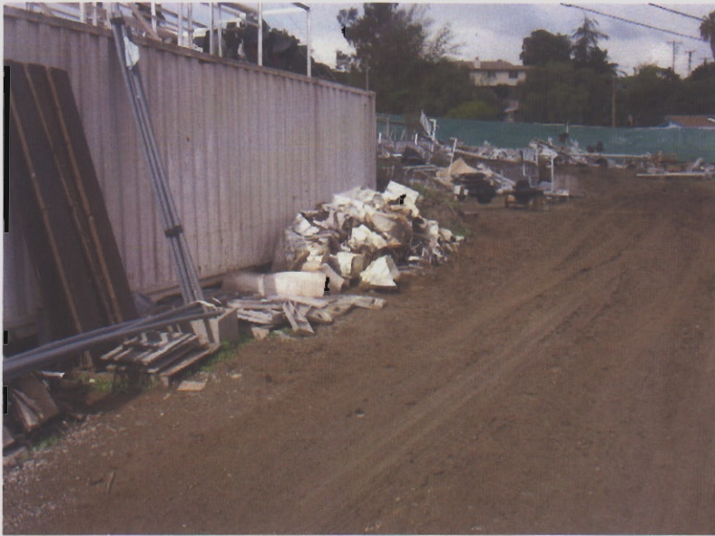
004. Although the trash containers were mostly empty in photo 003, trash is stored outside without cover or containment.
