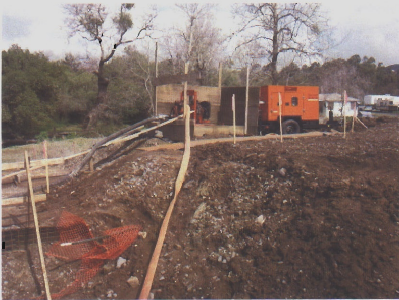
027. Groundwater dewatering for bridge work.
