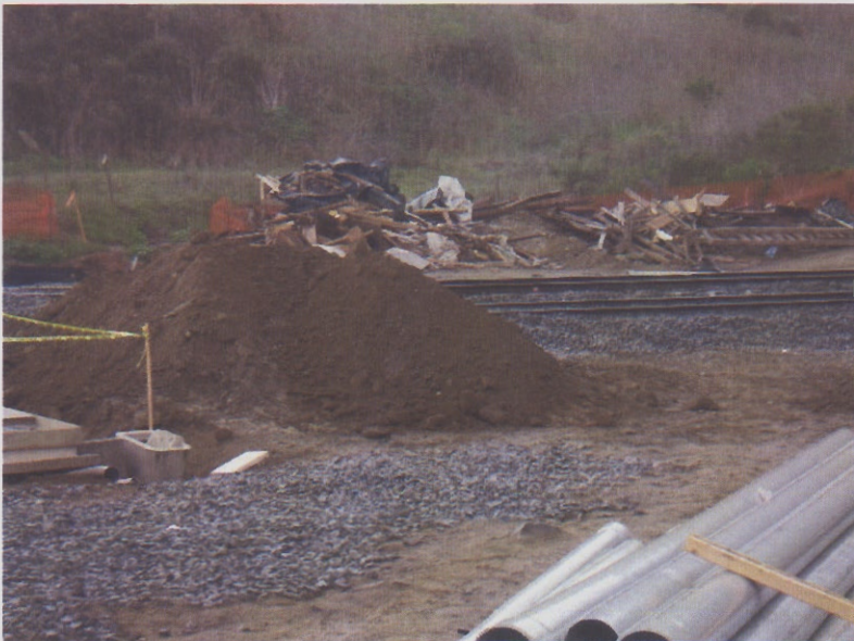
8. Soil stockpile has no cover or perimeter protection. Construction waste in the background has no cover or containment to minimize exposure to storm water.
