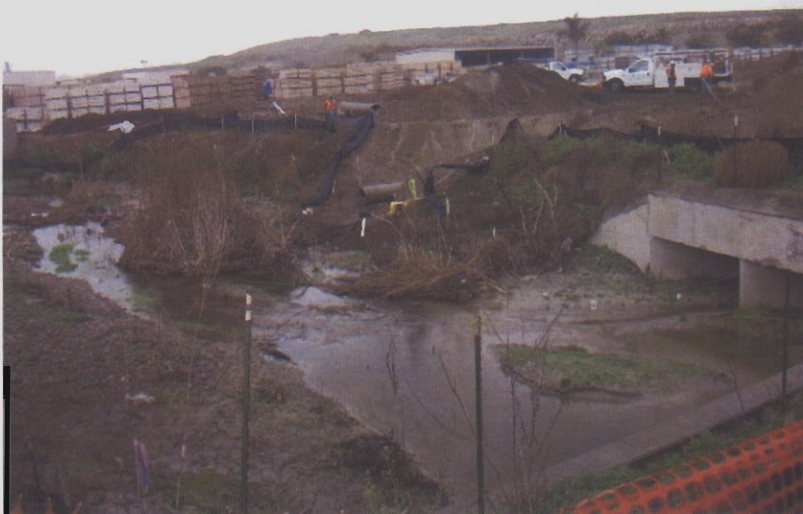
9. Construction work near the creek with inadequate sediment controls. Silt fence was removed around the pipe construction.
