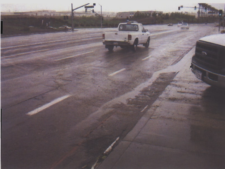
12. Sediment tracking onto Oceanside Blvd.
