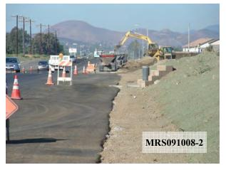
Scott Rd looking West, North side of road with hydroseed applied to 2:1 slope Note: stock pile removal.
