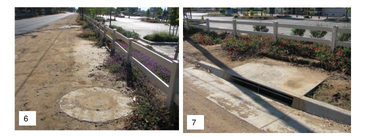
Photos 6 and 7 – Photos show the storm drain inlet along Palomar Street next to the parking lot. This inlet also appeared to not have any inlet filters or other treatment devices.
