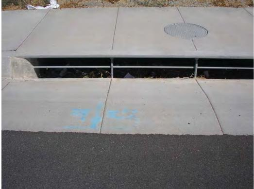
Figure 12. Storm Drain Inlet—no signage
