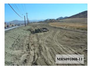
Excavated area south of Scott Rd. where drainage pipe and planned rip/rap will be applied. Looking East
