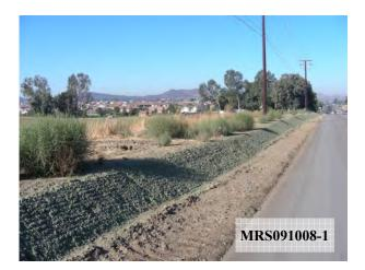
Scott Rd looking West, South side of road with hydro-seed applied to 2:1 slope
