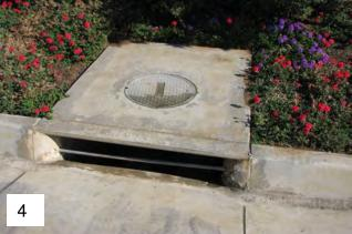
Photos 1 to 5 – Photos of the four inlet drains in the parking lot. None have inlet filters or other treatment devices.
