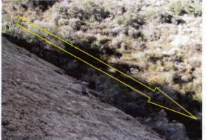
Photo 07: Shows flow direction and significant sediment loads sidescaped into natural waterway
