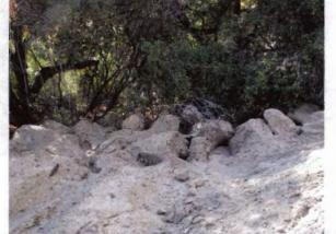
Photo 15: Sediment, silt and rocks are sidescaped into riparian corridor just downgradient from middle sediment basin
