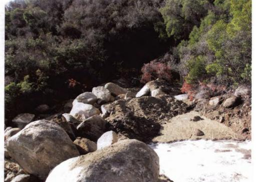
Photo 17: BMP (sediment basin) is placed within a natural waterway. Native riparian vegetation is destroyed by rocks and excavated dirt, impacting ecosystem.
