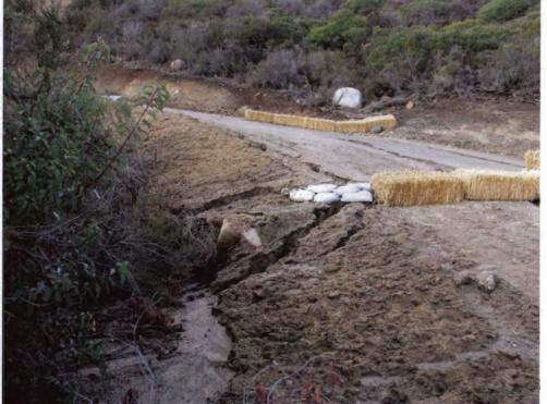
Photo 07: Inappropriate BMPs (hay bales and sand bags) are unable to contain and abate the high, concentrated flows causing rills and gullies.
