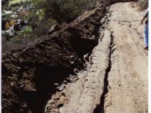
Photo 14: Looking downhill along access road shows erosion gullies
