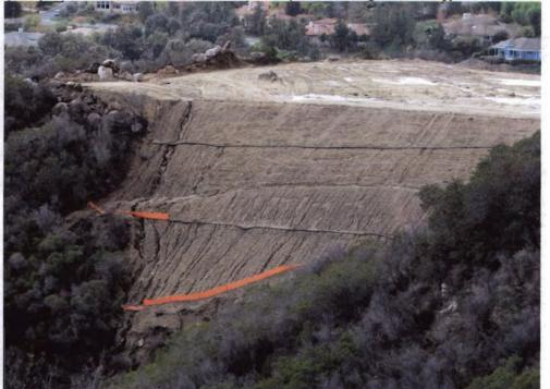
Photo 19: Failed BMPs on slopes; silt fence does not follow contour.
