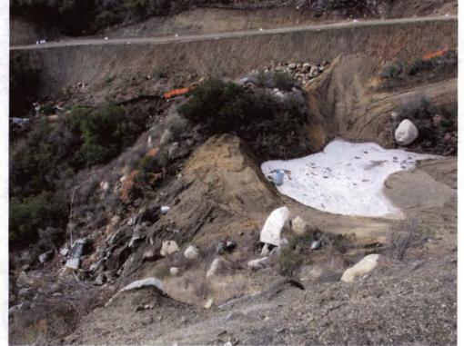
Photo 21: Third basin is built in a natural waterway or water of the State. Flow from this basin connects with the previous basin shown in photo 17.
