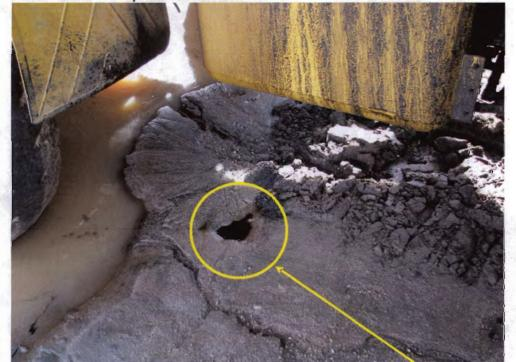
Photo 28: Construction vehicles are improperly stored with no drip pans to capture spill or leaks.
