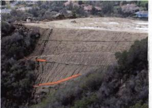
Photo 21: Close-up of erosion rills on slope shown in photo 20
