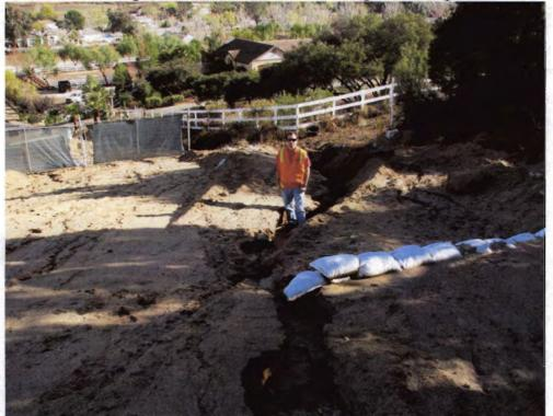
Photo 08: Erosion gullies were caused by high, concentrated storm water flows and failed BMPs.
