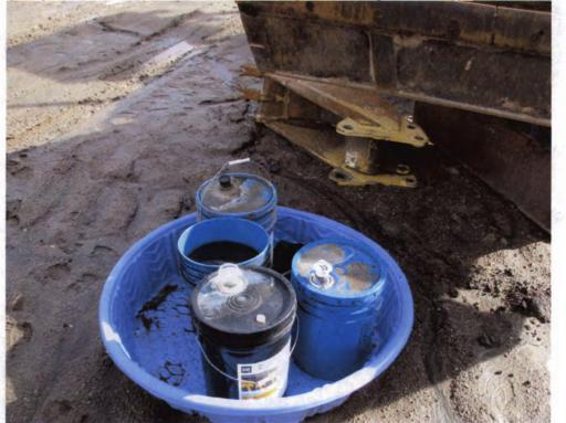
Photo 27: No BMPs to minimize exposure of mechanical construction wastes to stormwater or to potential accidents.
