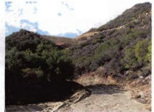
Photo 20: Shows inside and outside slopes (in fore and backgrounds) lack the proper BMPs to reduce erosion
