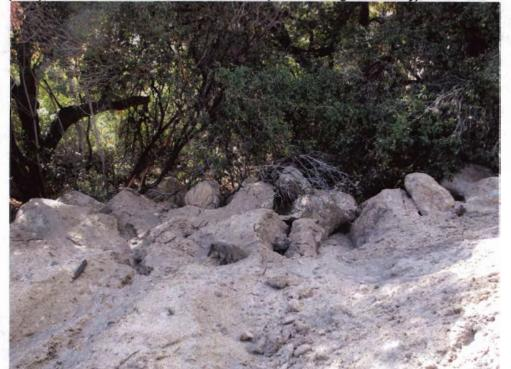
Photo 15: Rocks and dirt are sidescaped into a natural waterway (Water of the State). Discharge is to the hardened channel flowing to Bear Creek.
