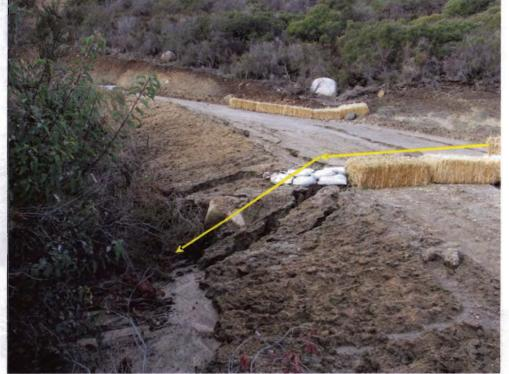
Photo 20: The road was constructed (w/o proper permit) directly across a natural waterway. Erosion effects can be seen across the road.
