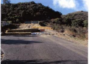
Photo 01: Site entrance at Claremont Street shows inadequate BMP to prevent erosion
