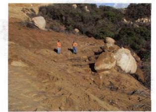
Photo 11: Construction fill (sediment, silt, rocks, and boulders) dumped in waterway (two inspectors are standing waterway)
