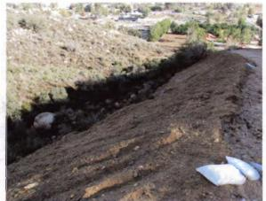
Photo 08: Outside slope not stabilized, discharge of fill (rocks, boulders, and vegetation) in waterway
