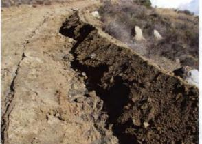
Photo 13: Shows severe erosion along access road leading to middle basin
