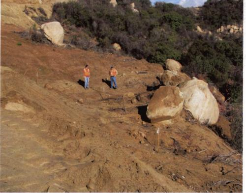
Photo 13: This area lacks erosion and sediment controls as significant quantities of dirt is placed alongside a natural waterway.
