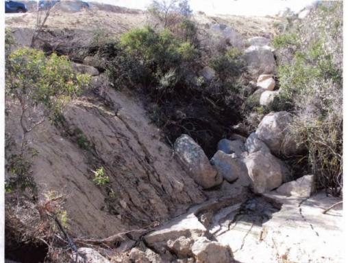
Photo 11: Rocks and boulders were sidescaped into the natural drainage area along the fire road. The caked sediment is evidence of flow blockage.
