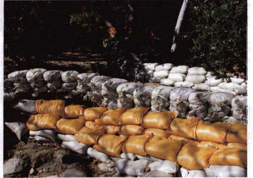
Photo 24: Fill in a natural waterway or water of the State is used as a BMP.
