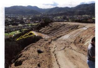
Photo 09: Unstabilized slopes and access road, breached sediment basin allowed sediment discharge (insert) in waterway
