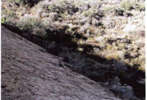
Photo 10: Evidence of recent grading of the fire road shows graded dirt was sidescaped down embankment towards natural waterway.
