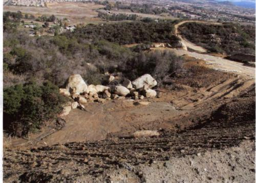
Photo 22: More fill of rocks and excavated dirt were sidescaped into natural waterway.
