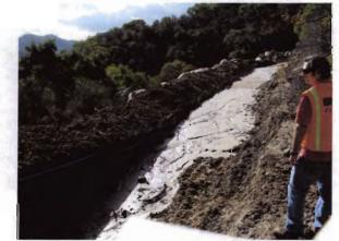
Photo 17: Shows significant sediment and silt in sediment basin
