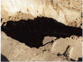
Photo 10: Failed slope along access road
