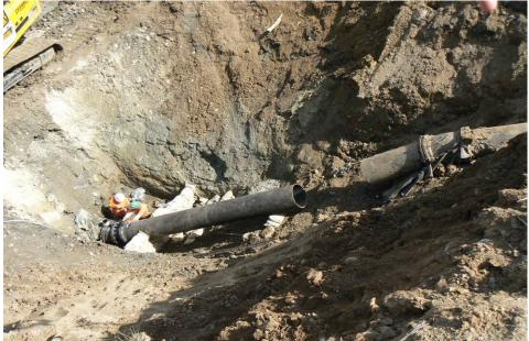
Figure 8. Force main rupture repair work on March 26, 2010
