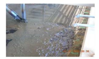
2009 View of Cooling Tower basin during maintenance outage, tank basin was allowed to settle with all residual solids collected and hauled offsite for disposal. This BMP for facility was mandated by the City of Escondido after investigation 2008 violation for TSS.
