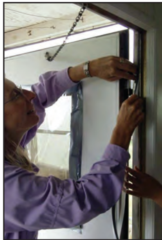
A Viva Verde contractor installs weather stripping to the door frame of a southern New Mexico home.
