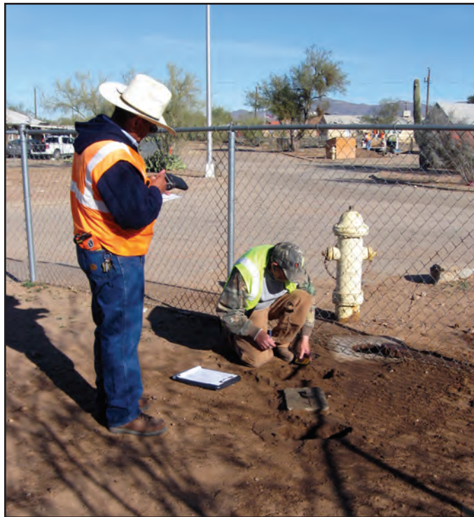
Utility workers in Sells, Arizona, plot the location of a water main, a practice known as "potholing."
