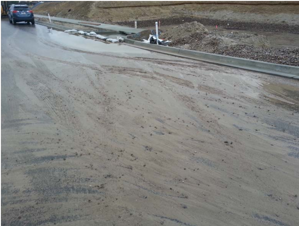
Figure 2. May 8, 2015, Sediment Discharge. View of sediment in street (Orlando Drive) after storm event. Photograph taken by Frank Melbourn, San Diego Water Board. 20150508_191716.jpg
