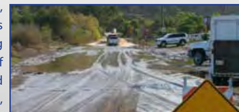
Flooding along Hollister Road in the Valley
