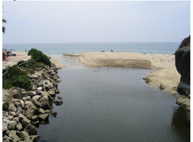
Figure 2. Example of ocean outlet maintenance activities. Looking from Coast Highway. Note the channel cut in the sand berm. Photo taken July 26, 2006.
