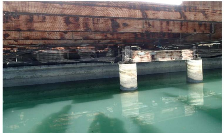
Wooden deck support members to be replaced are located above the highest high tide and would be removed and replaced from above after removal of the top epee decking planks. No work in the water is
