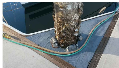
TYPICAL TRIANGLE FRAME PILE GUIDE ④
