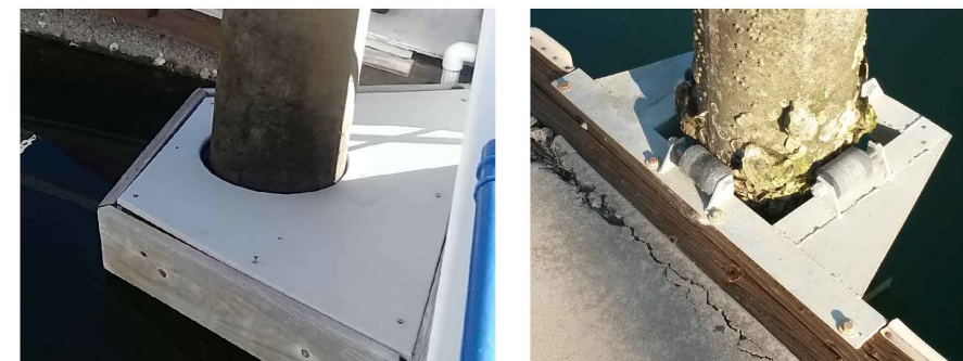
TYPICAL SIDE PILE GUIDES ⑨
