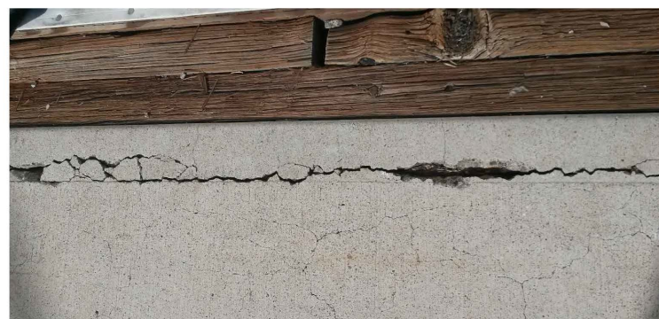
TYPICAL EDGE CRACKING 2 ③ SCALE: NTS
