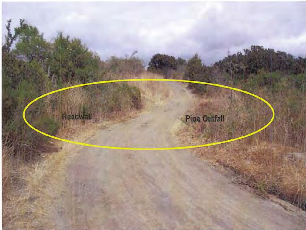
Figure 1. North-facing overview of road repair location.
