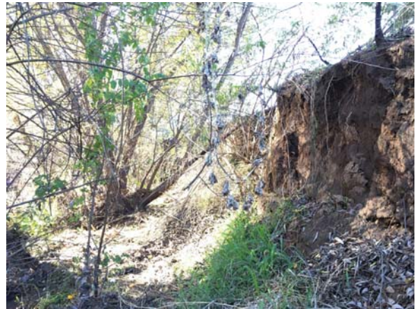
Figure 3. View of right bank at XS2 looking downstream showing highly erodible streambanks typical of the assessment reach.
