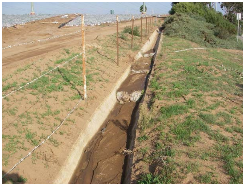
Figure 5. Use of Sandbags near Strawberry Fields, Cannon Rd. near Interstate 5, Carlsbad Watershed.
