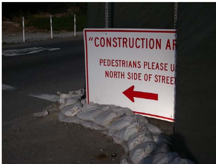
Figure 4. Use of Sandbags upstream of Moonlight State Beach, Encinitas Blvd., Carlsbad Watershed.
