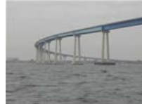
San Diego Bay Bridge
