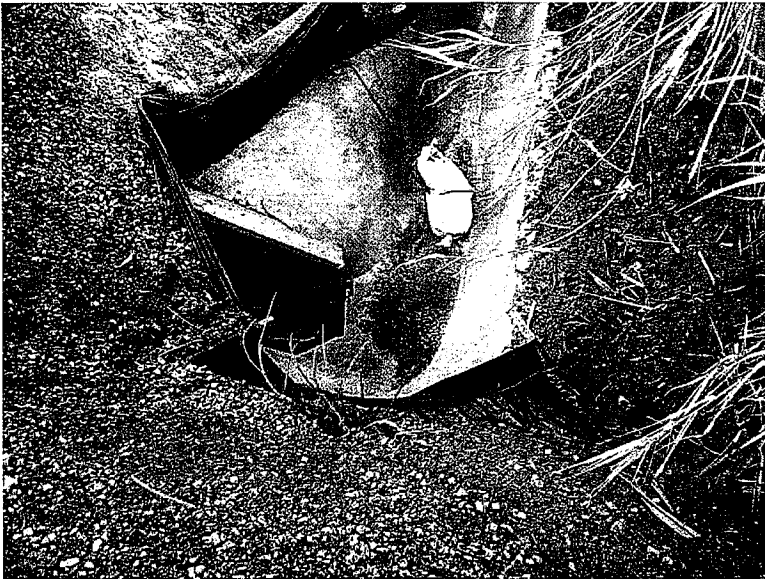
13. This photo was taken at the Escondido Avenue Station in the City of Vista. Silt fence has failed around this inlet at the north east corner of the station. Sediment and off color water was observed in the storm drain culvert. Photo looking east.
