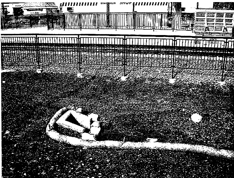
24. A storm drain inlet has inadequate protections. The soil and slope around the inlet did not have erosion controls or soil stabilization. Photo looking North.
