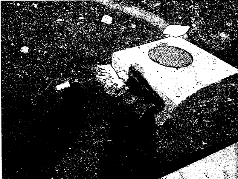
32. A closer view of the inlet in photo 31 shows that storm water flows had previously overtopped the gravel bags resulting in a discharge of sediment. Photo looks North east.
