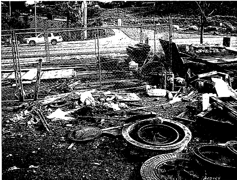
8. Construction trash left out at the yard without cover or containment to prevent contact with storm water. Photo looking North.
