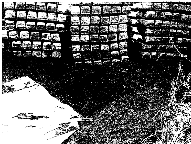
6. The plastic lined channel begins at this point receiving storm water flowing beneath the stockpile of concrete railroad ties. Photo shows channel erosion occurred beneath the railroad ties. Photo looking South.
