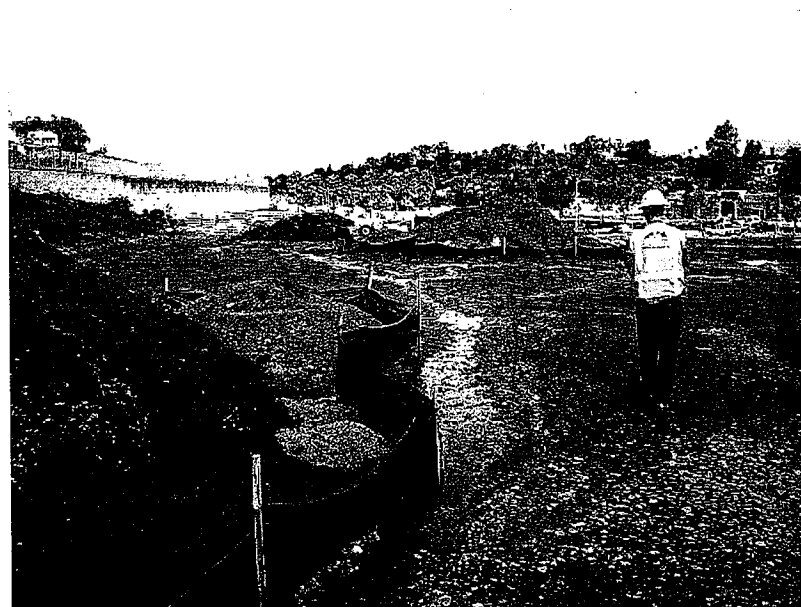
12. Runoff from the culvert in photo 11 flows through the bare dirt in the construction yard to the plastic lined channel in photo 1. Photo looks West.
