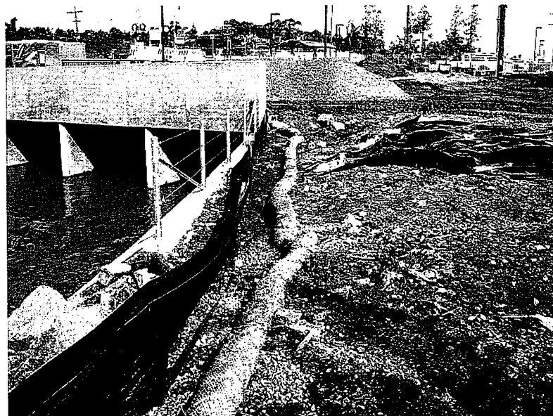
27. Sediment flows between the fiber roll and the silt fence were not held back. Silt fence is not properly implemented. Photo looking east.
