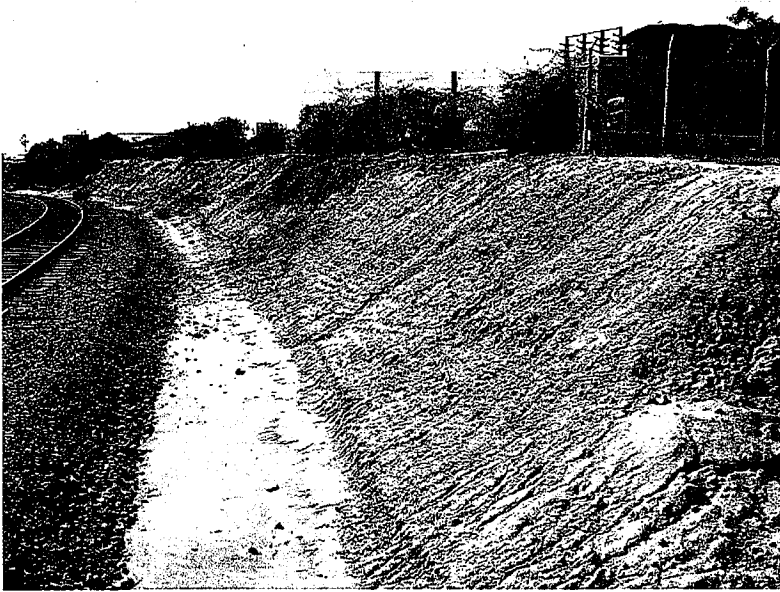
34. Slopes are without sediment or erosion controls. This area is south west of the parking lot. The slope is north of the track going southwest to intersect the Coaster track. Photo looking West.
