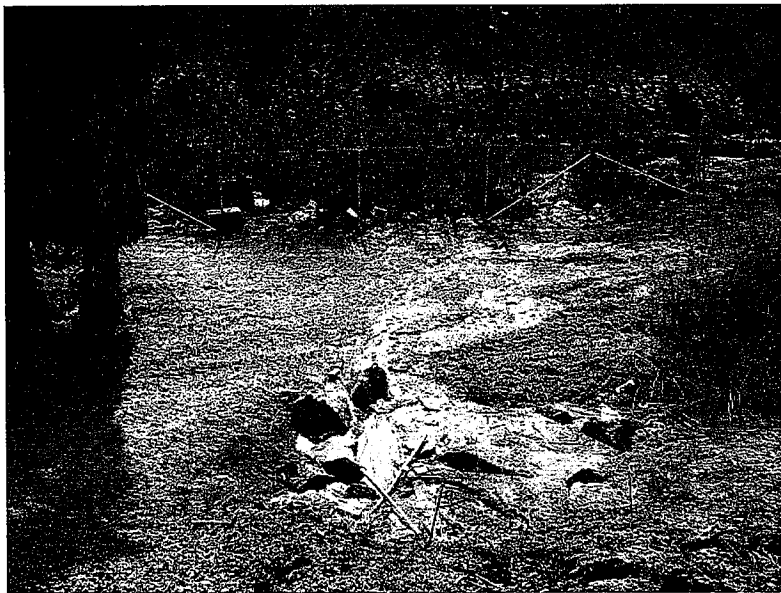
23. A storm drain outfall farther west from the gully in photo 17. This outfall shows evidence of sediment discharged from the Melrose Station to Loma Alta Creek. Photo looking South.
