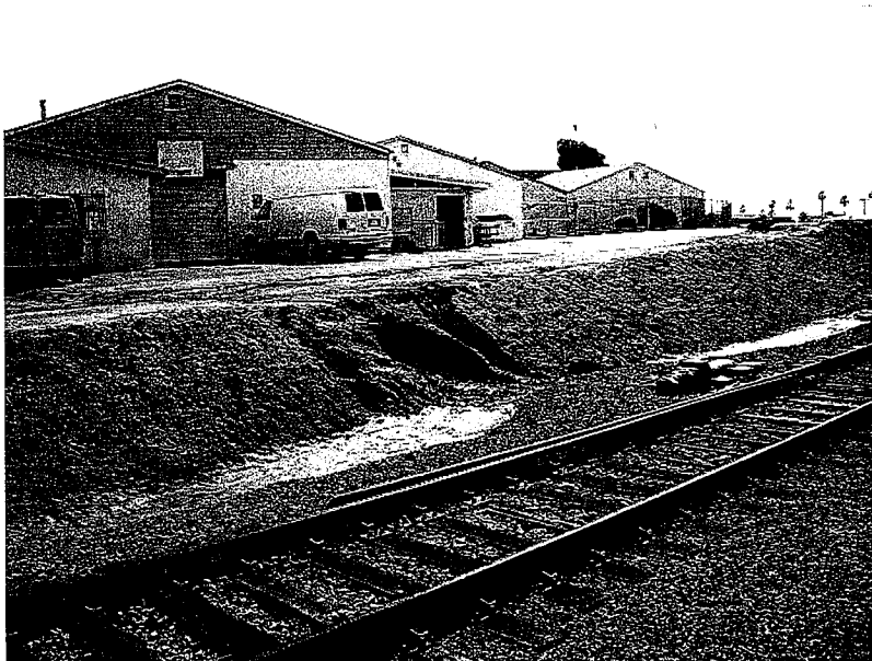
35. Slope with significant erosion has exposed the underground utilities.
