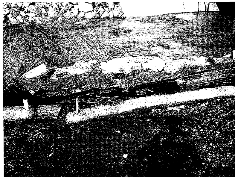
30. The sheet flow in photo 27 carries sediment and overwhelms the improperly implemented and maintained fiber rolls and silt fencing. Sediment discharged to Loma Alta Creek. Photo looking North.
