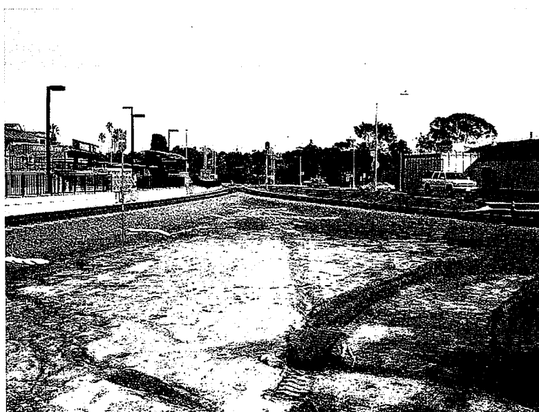
36. The area between the tracks has some chevrons of gravel bags implemented. Photo looks east.
