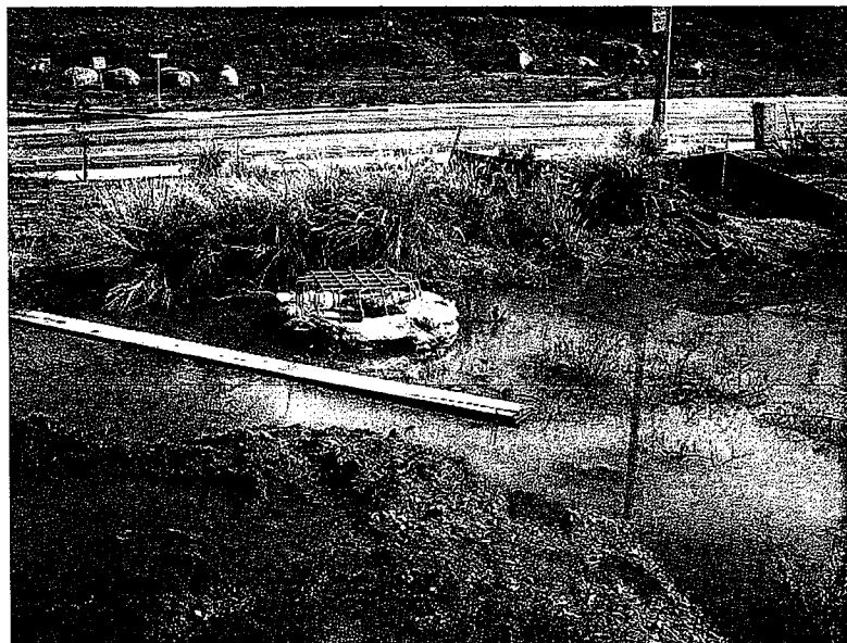
9. Second inlet within Mar Vista Storage Yard. Water did not appear to flow into this inlet but rather pooled here and then flowed across the construction yard to the inlet in photos 3, 4, and 5. Photo looks North.
