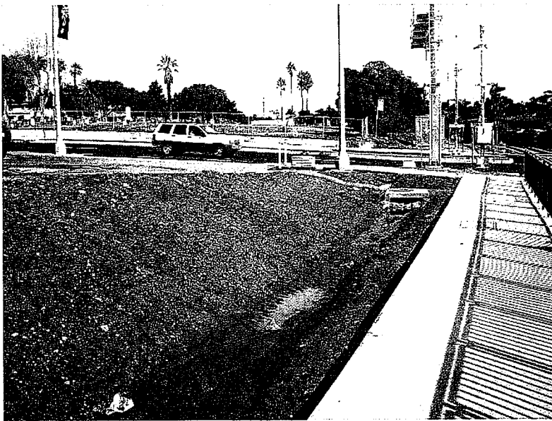
31. Exposed soils with no erosion or sediment control lead to a storm drain inlet. This was located north of the tracks next to South Coast Highway. Photo looks East.
